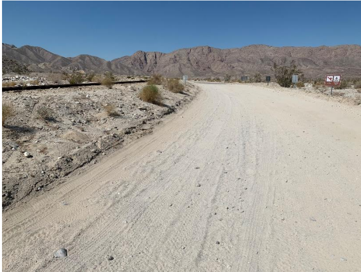
Photo 13: Southwest facing view of the new waterline alignment along USG railroad tracks.
