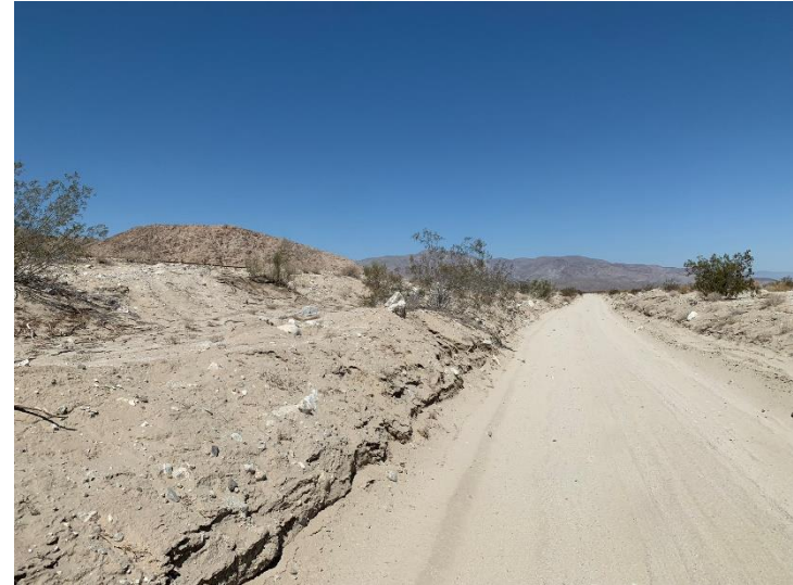
Photo 14: Southwest facing view of the new waterline alignment along USG railroad tracks.
