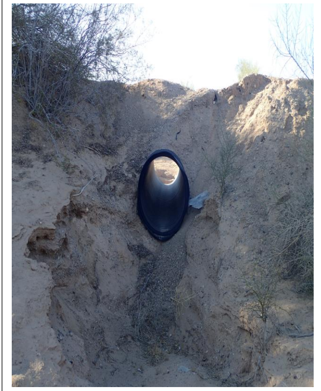
17. Pipe from wash to north side of SR 78 on southeast portion of site
