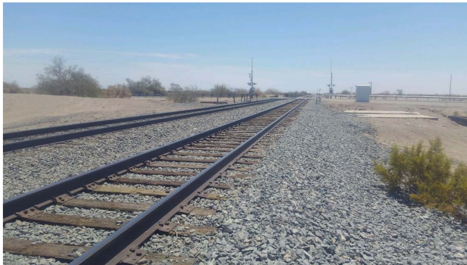
Figure 6. Overview of IMP-3424 facing southeast toward State Highway 78.
