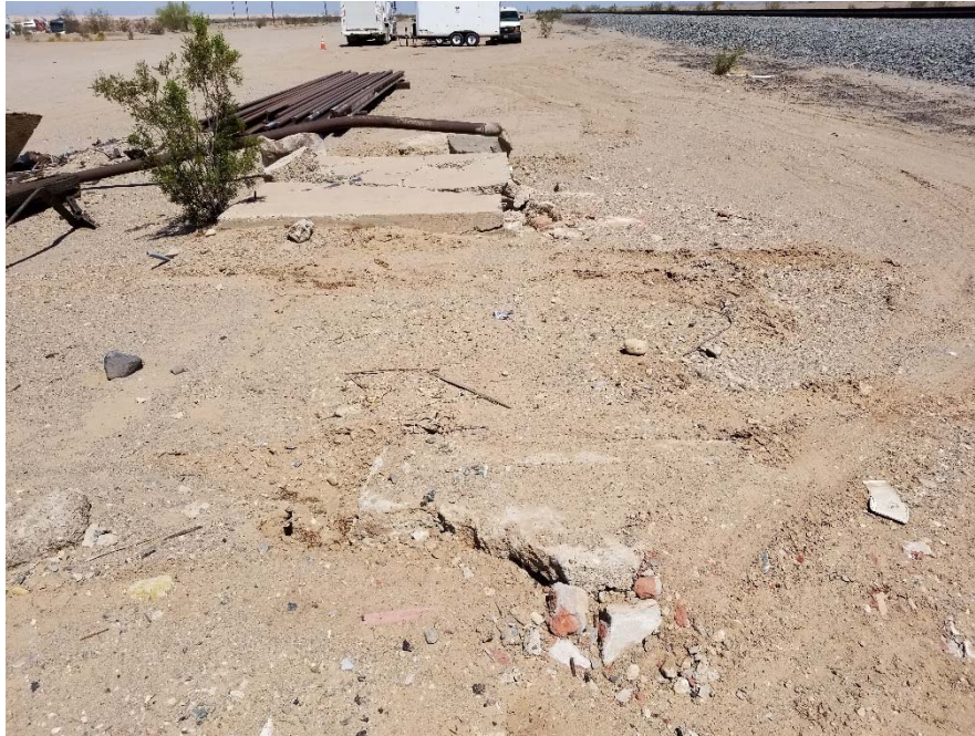
Figure 9. IMP-8634H overview facing northwest.
