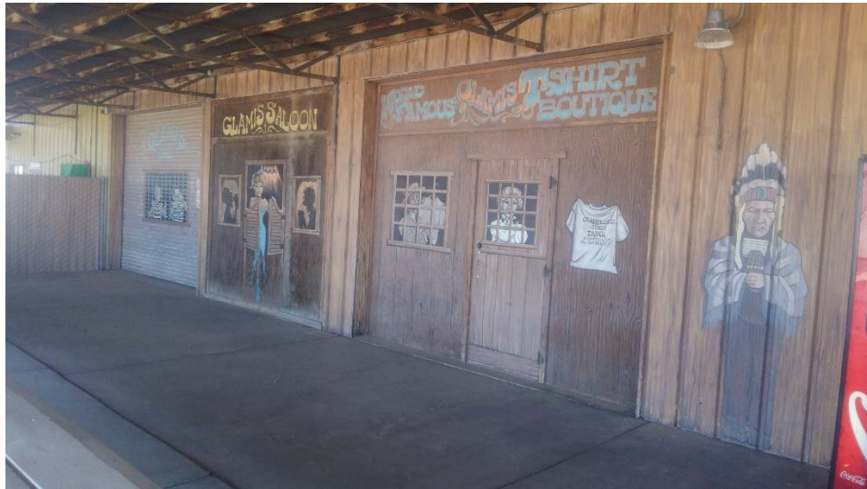
Figure 14. Glamis Beach Storage decorative painting at front porch, view to east.
