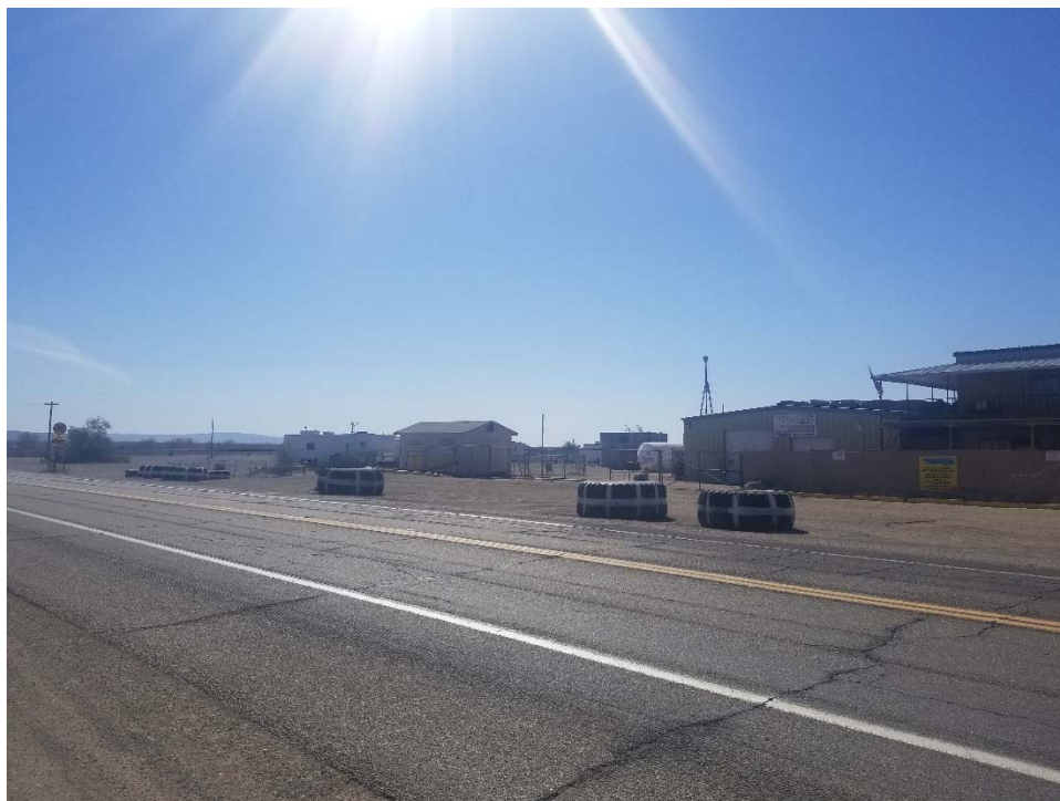
Figure 16. GSP-KM-S-3/Highway 78 at Glamis Beach Store complex, surface cracks, view to east.
