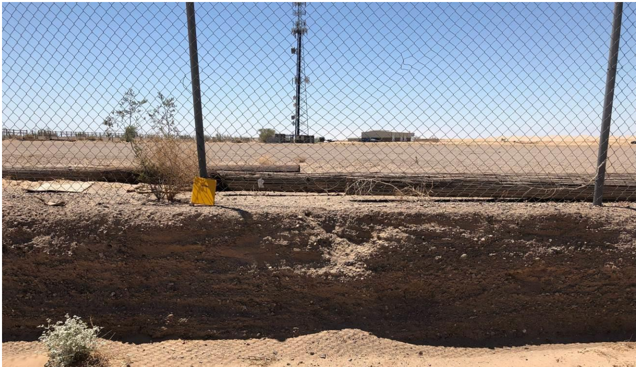
Figure 3. Previously graded pad built of undocumented gravel fill. Photo taken just south of the intersection of SR 78 and the UPR, looking south at the radio tower located in the southeastern corner of the study area.
