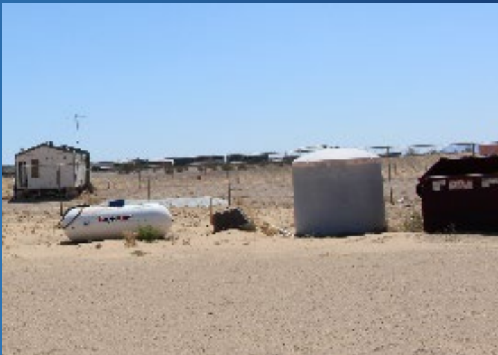
Dilapidated pre-fabricated residential structure
