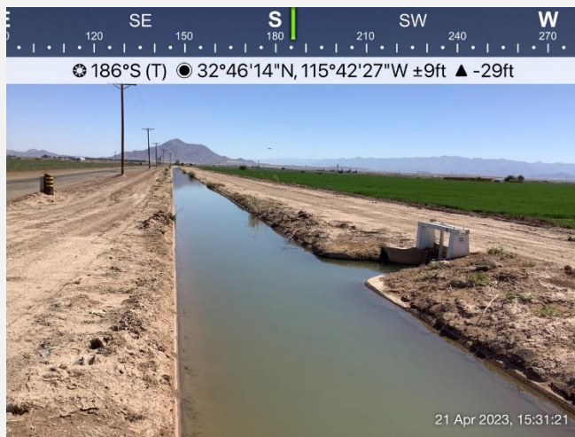
Photo Point 1. A larger concrete irrigation ditch that runs north/south and eventually connects to the Westside Main Canal (Photo Point 14) and may be jurisdictional.
