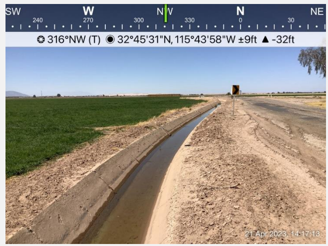
Photo Point 10: A wetted concrete irrigation ditch. This ditch runs north/south for a short distance adjacent to the agriculture area it conveys water to. This ditch is closed and likely non-jurisdictional.
