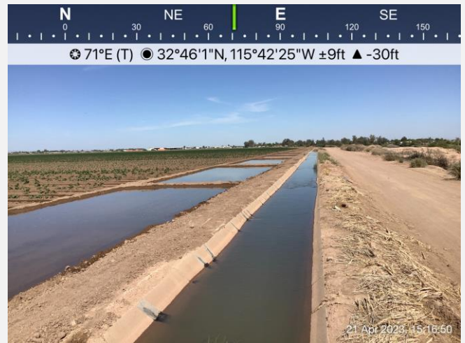
Photo Point 4: View of wetted earthen irrigation ponds adjacent to a smaller concrete ditch that may be jurisdictional, as it receives water from the larger Fig Canal.
