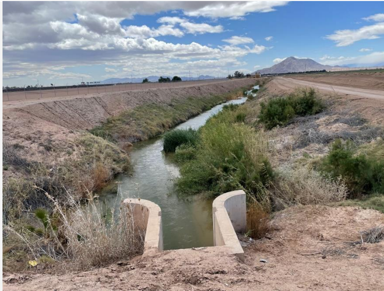
Exhibit 26. View of the Fig Drain and an intact concrete weir near Diehl Road, facing south.
