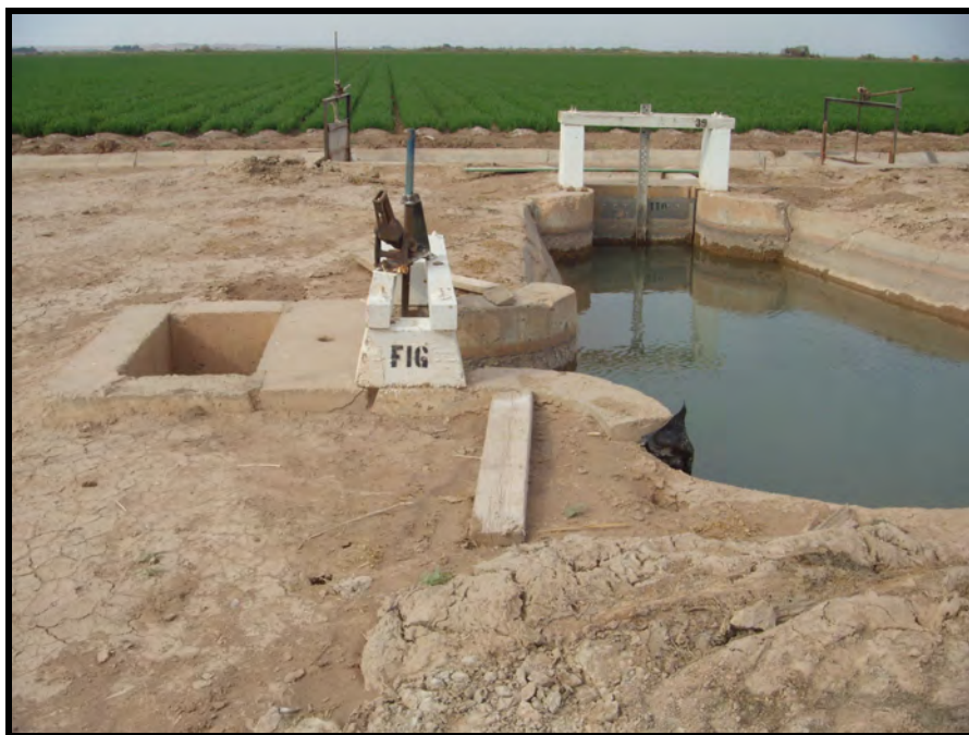
View of culverts and gate structures located in portion of canal north of Evan Hewes Highway
