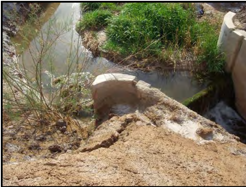
View of south culvert with drop structure
