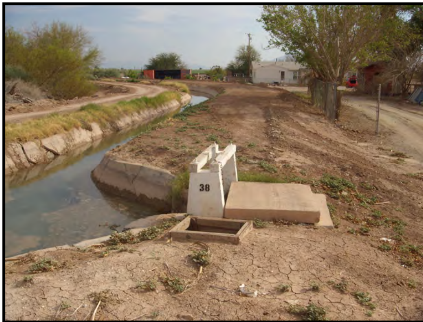
View of gate structure and turnout in canal south of Evan Hewes Highway
