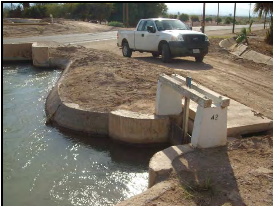
Wing culvert and gate structure on the west bank north of Evan Hewes Highway
