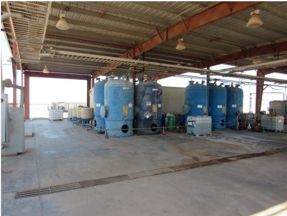
**Photo 40: Looking within the southern portion of the ES Mineral Test area at various liquid containers/tanks. The blue tanks are all labeled empty. Containment curb around this area and floor drains that are connected to the brine pond.**
