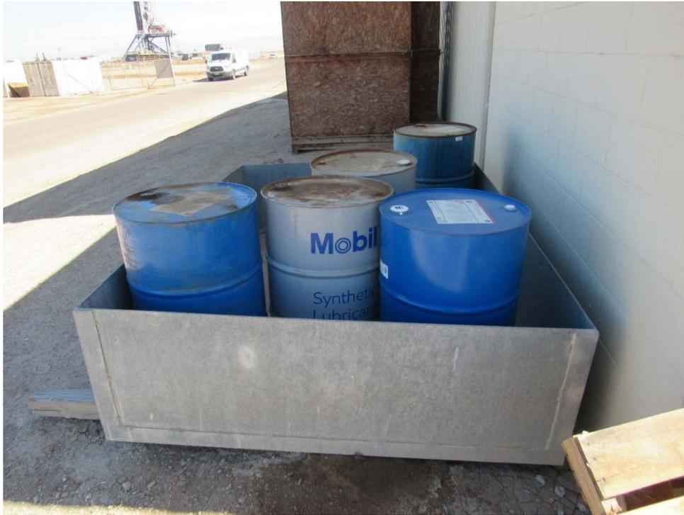
**Photo 15: Looking at a temporary secondary containment bin along the west wall of the secondary containment area from Photo 11.**
