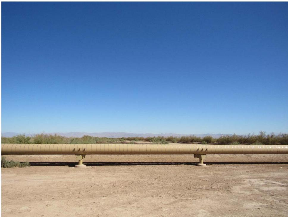
**Photo 80: Looking at the geothermal pipeline that extends from the geothermal plant to the well pads.**
