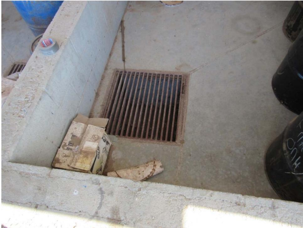
**Photo 13: Looking at the sumps that are inside the secondary containment from Photo 11, these drain to the brine pond.**
