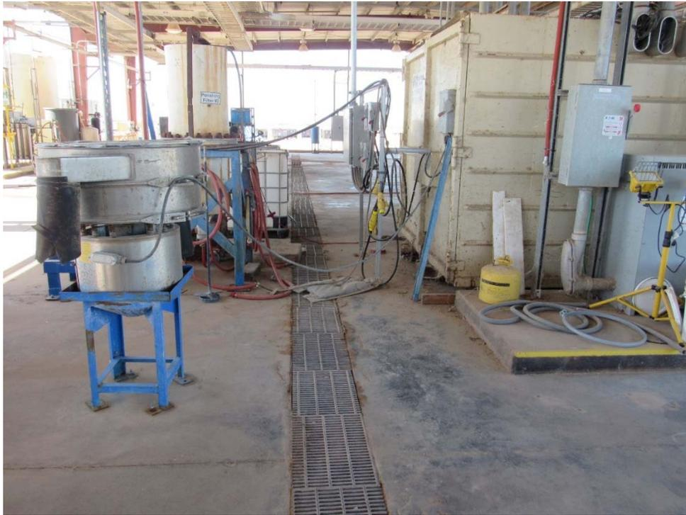
**Photo 43: Looking at the drain within the ES Mineral Test area that drains into the brine pond.**
