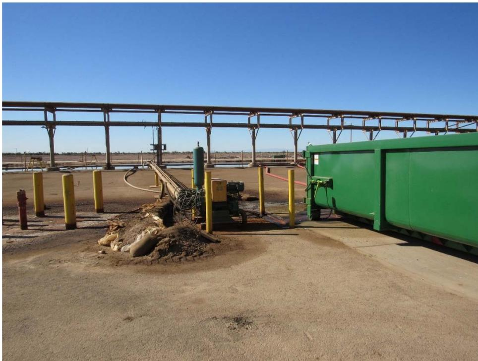
**Photo 59: Looking at the sump on the north side of the brine pond. The area had recent leakage of brine during extraction into green bins, all contained and sump pumped back into brine pond.**
