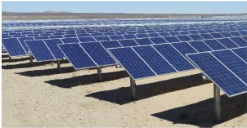
Typical Single-Axis Tracking Solar Panels
