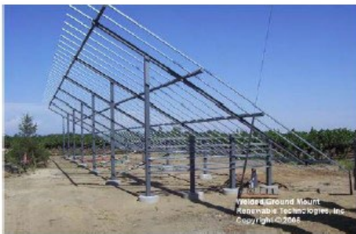
Typical Fixed-Tilt Mounting Structure
