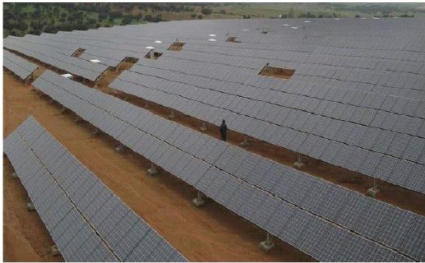
Typical Fixed-Tilt Solar Panel Rows
