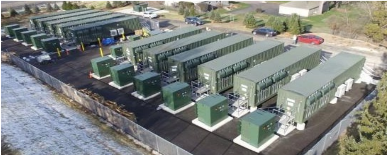
Modular BESS Installed on Concrete Pad
