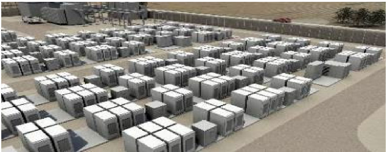
Modular BESS Installed on Multiple Concrete Pads
