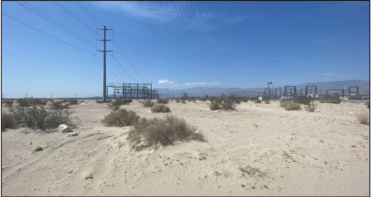
Photo 1: View of the project footprint looking south towards existing Ramon Substation, showing disturbed Creosote Bush Scrub habitat.
