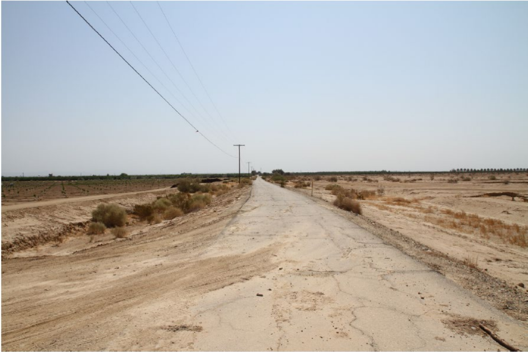
Figure 3.2-3. Key View 2: View from Garvey Road, Looking East
