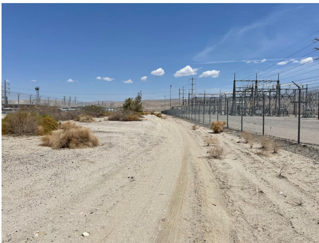
Photograph 2. Project Area west of the Ramon Substation, facing north.
