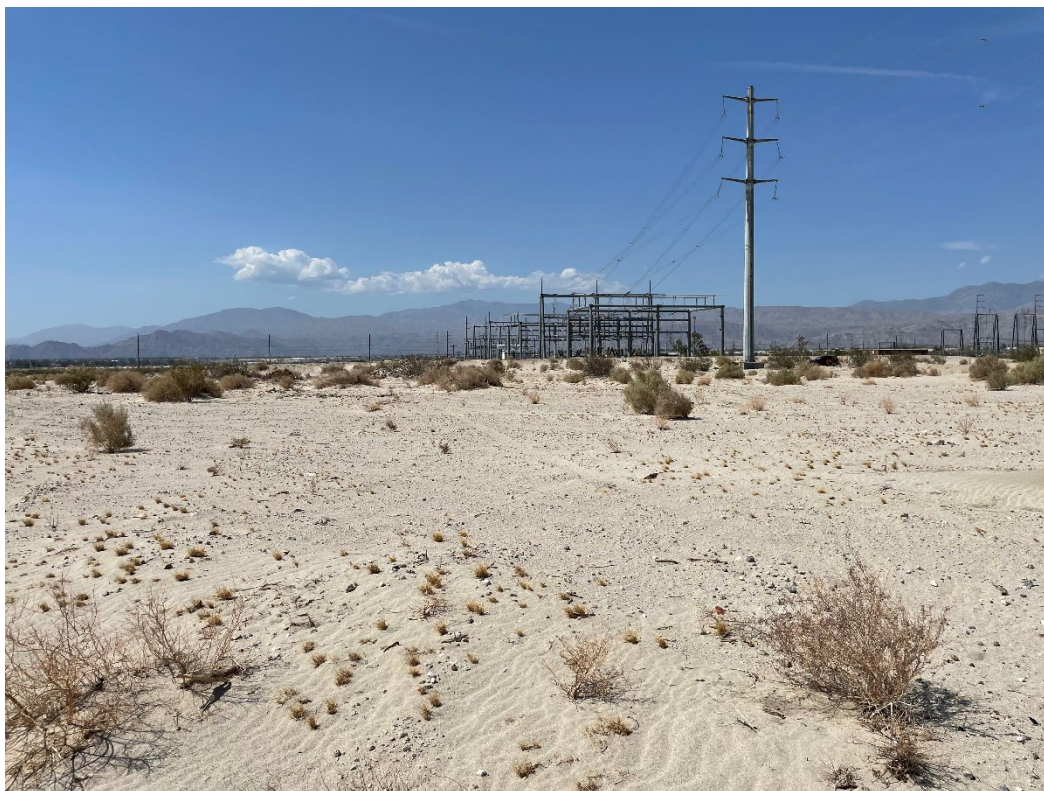
Photograph 5. Project Area north of the Ramon Substation, facing south.
