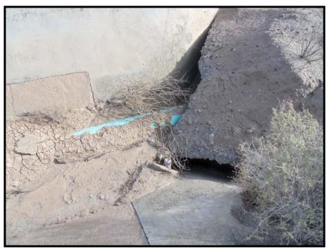
Photo 13: Subject site looking at a section of pipe buried in the concrete lined ditch, which delivers raw water to the Imperial Lakes development.
