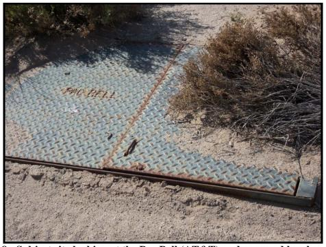
Photo 8: Subject site looking at the Pac Bell (AT&T) underground box located on the southern boundary of the site, the line runs parallel to dirt road on north side of Even Hewes Highway.
