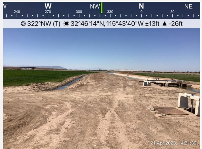
Photo Point 2: View of a smaller concrete and larger gated concrete ditch running parallel.
