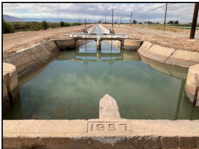
Portion of Dogwood Canal east of Pitzer Road showing concrete lining and check/drop feature with 1957 date stamp, facing east
