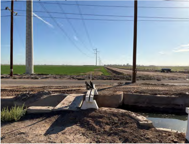
Portion of Daffodil Canal showing check/drop structure with Pfizer Road in background, facing east
