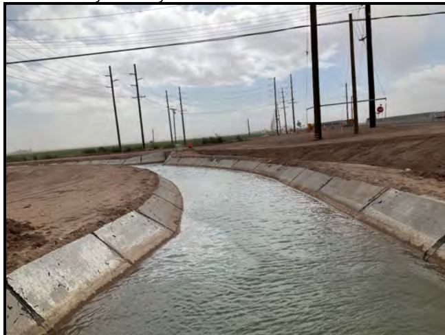
Portion of Dogwood Canal by Dogwood Road showing recently installed concrete lining, facing south
