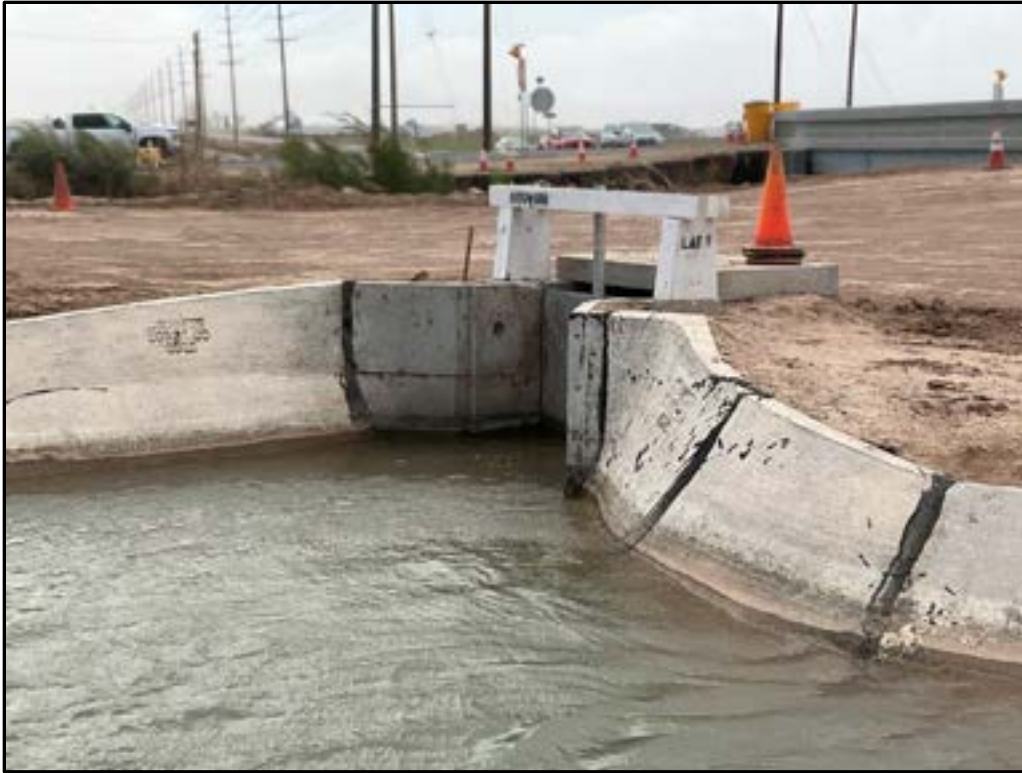
Figure 5-12. Portion of Dogwood Canal gate feature and concrete lining with date stamp, east of Dogwood Road, facing south
