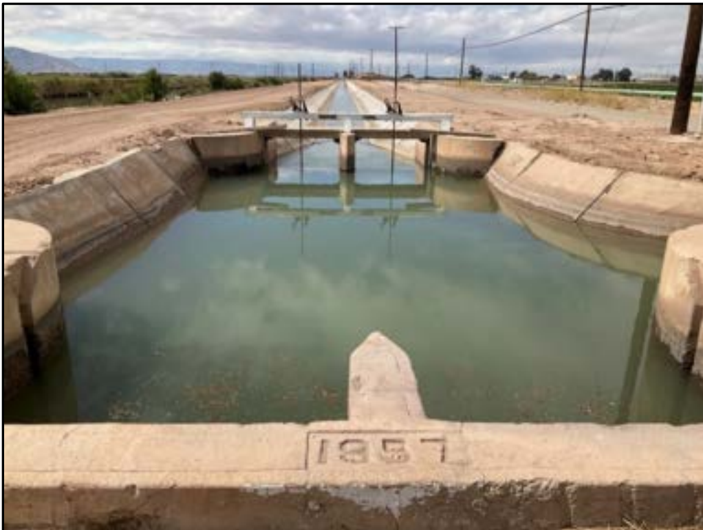
Figure 5-13. Portion of Dogwood Canal east of Pitzer Road showing concrete lining and check/drop feature with 1957 date stamp, facing east
