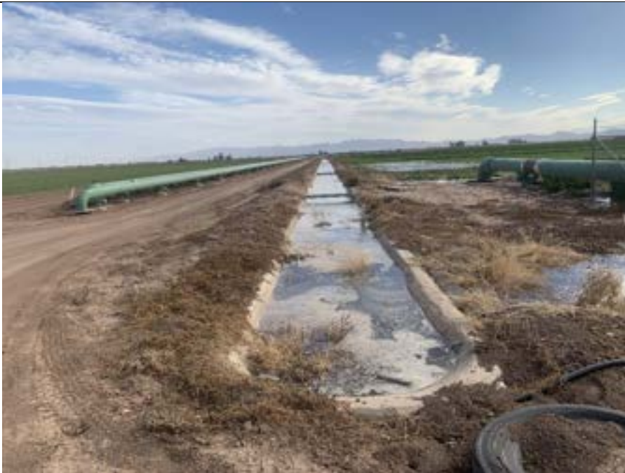
Photo 15: Concrete-lined v-ditch and existing pipeline, looking south. Proposed transmission line would be mounted to the green pipeline on the left side of the frame.
