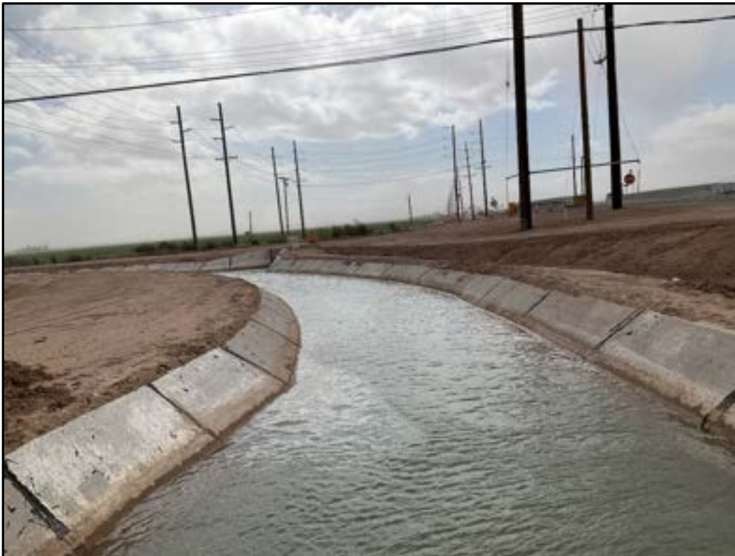
Figure 5-11. Portion of Dogwood Canal by Dogwood Road showing recently installed concrete lining, facing south
