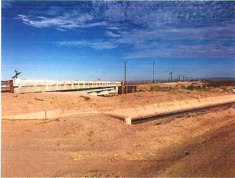
Photograph 1: Looking at the bridge from the southeast.
