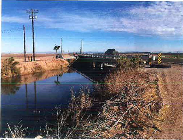
Photograph 6: West side of the bridge.
