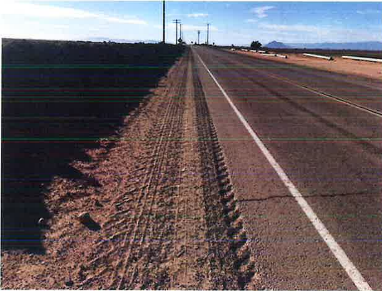
Photograph 10: Roadway on the north side of the bridge.
