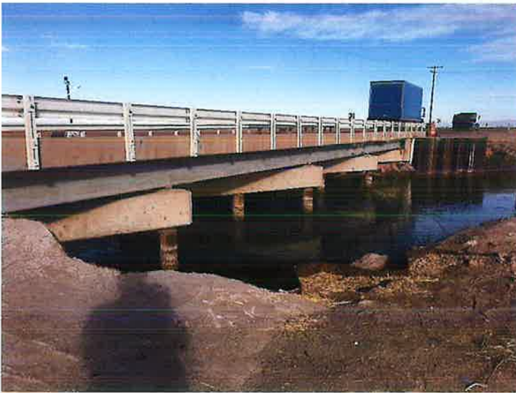
Photograph 2: Looking at the bridge from the southeast.
