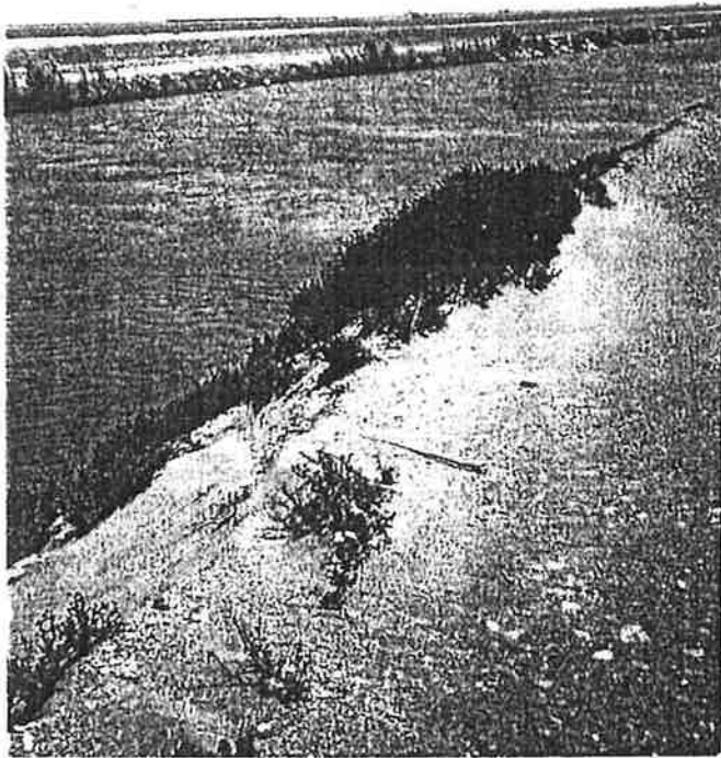
4/28/99 Westside Main Canal segment north of SR 98, looking NW.
