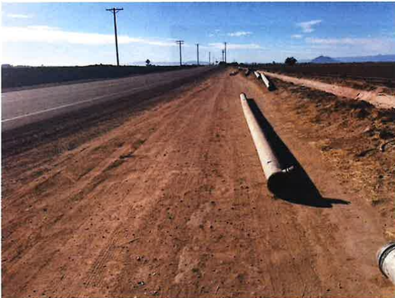
Photograph 9: Roadway on the north side of the bridge.
