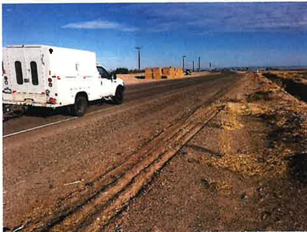
Photograph 4: Roadway to the south of the bridge.
