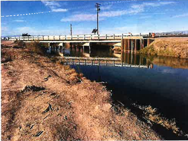
Photograph 3: Looking at the bridge from the east.
