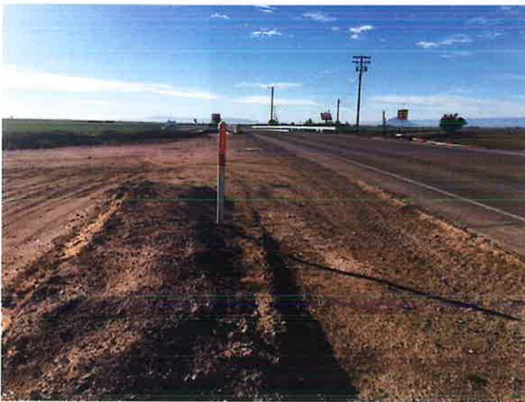
Photograph 11: Roadway on the north side of the bridge.
