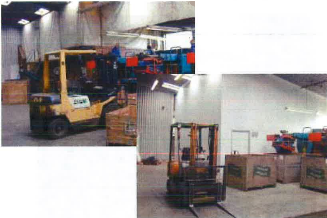
Figure 21 Old (left) and new (right) sound enclosures on onion grading line
