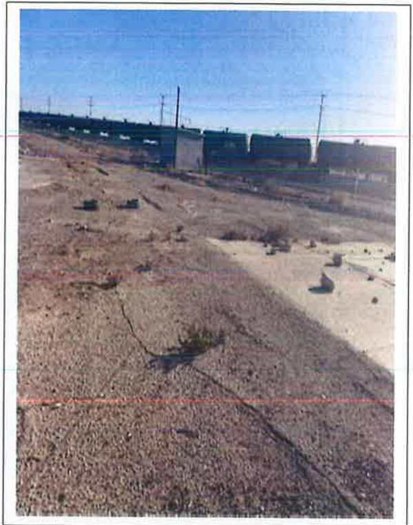
8. Old scale house; concrete pad; railroad tracks in background
