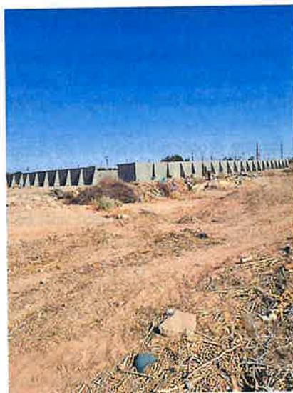
Photograph 2. Industrial Hemp Processing Facility (APN 057-010-052-000), A Structure Composed of Cinder Block and Concrete Walls and Pad, View Southeast
