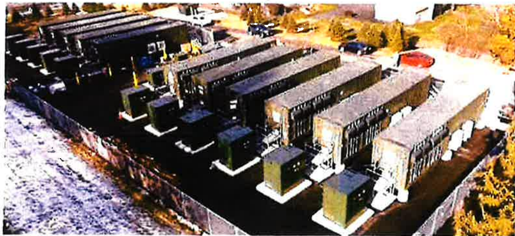
Modular ESS Installed on Concrete Pad
