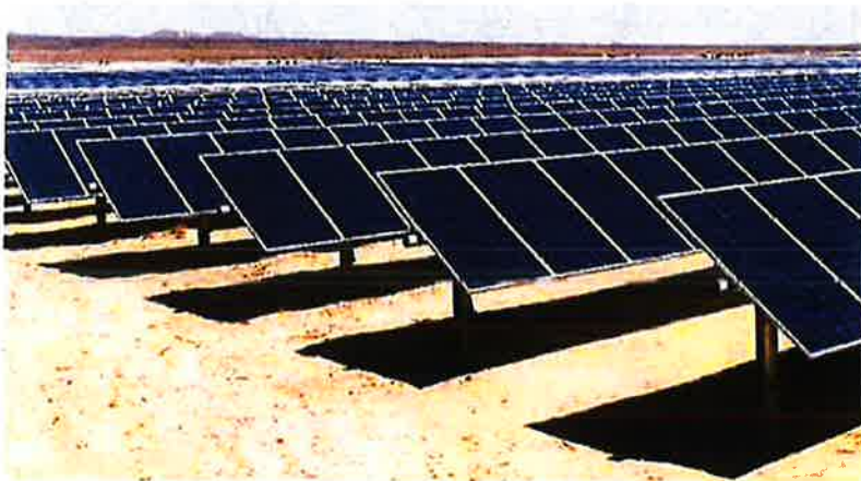
Typical single axis tracking solar panels
