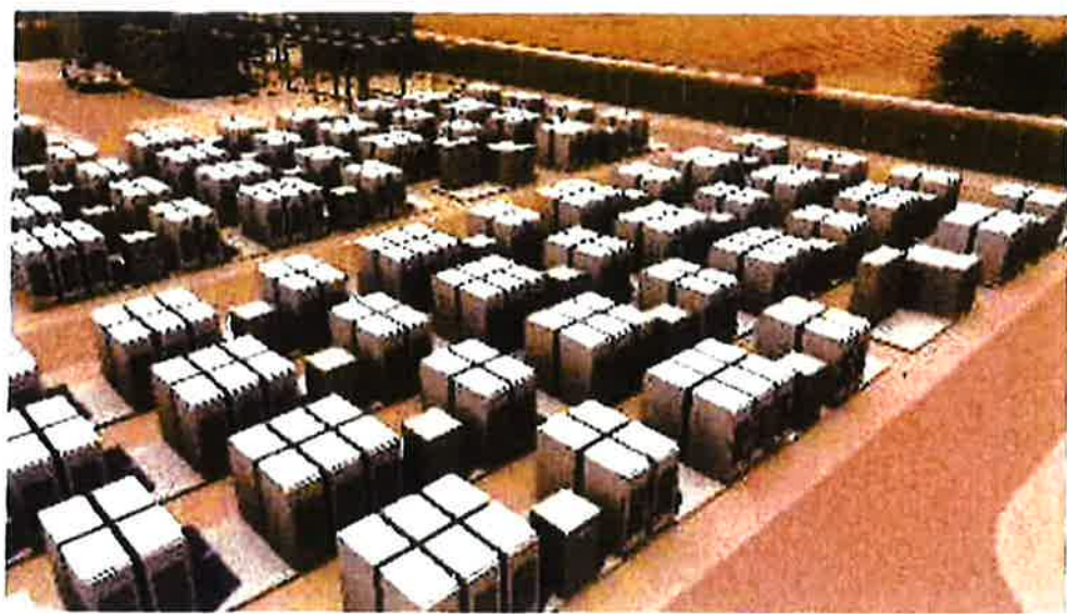
Modular ESS Installed on Multiple Concrete Pads
