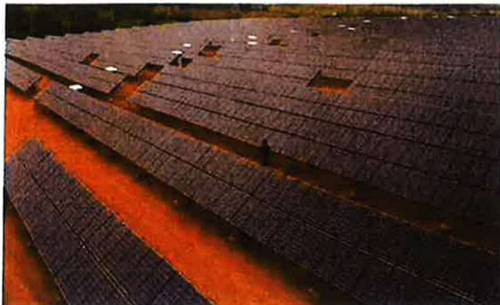
Typical fixed-tilt solar panel rows
