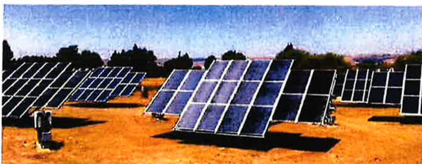
Typical dual axis tracking solar panels
