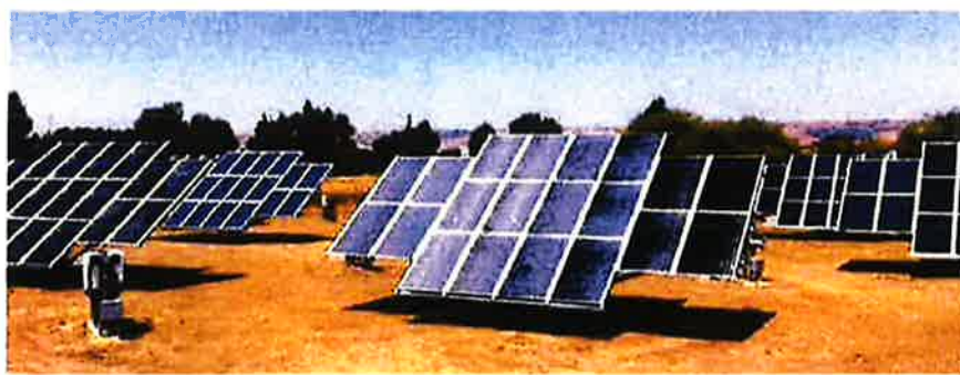
Typical dual axis tracking solar panels
