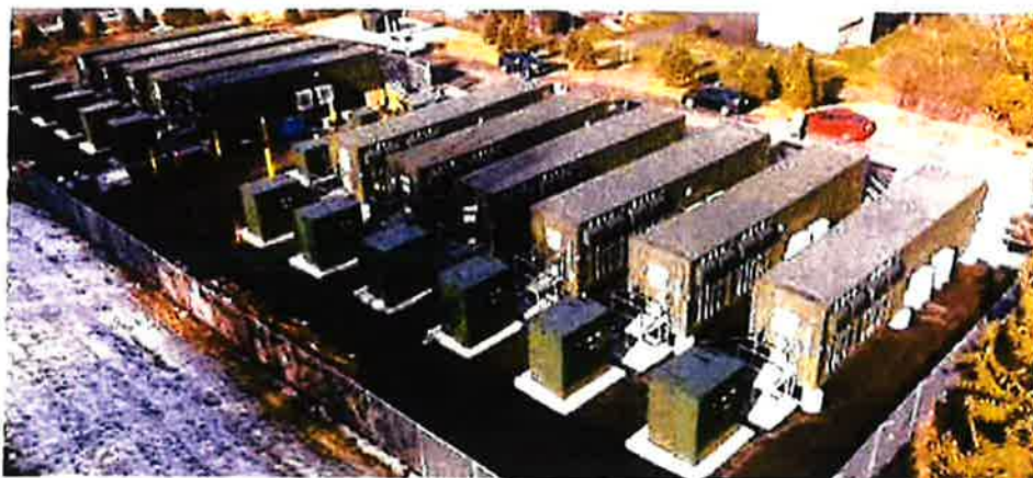
Modular ESS Installed on Concrete Pad
