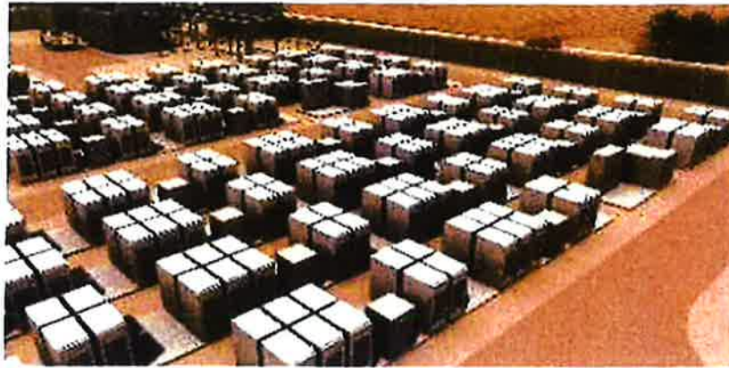
Modular ESS Installed on Multiple Concrete Pads
