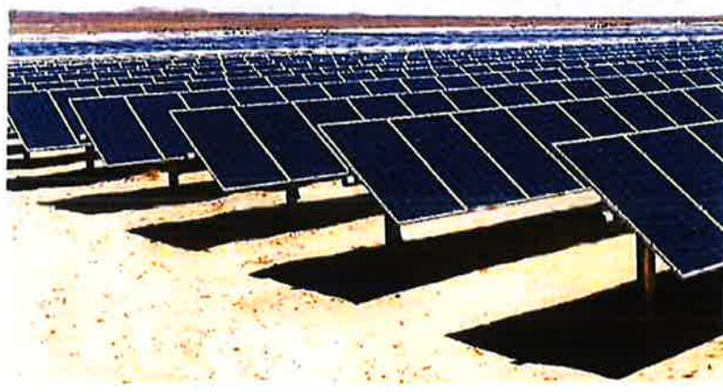
Typical single axis tracking solar panels
