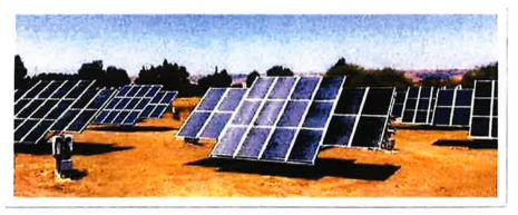
Typical dual axis tracking solar panels
