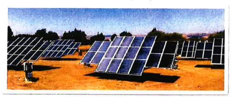
Typical dual axis tracking solar panels
