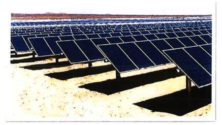
Typical single axis tracking solar panels
