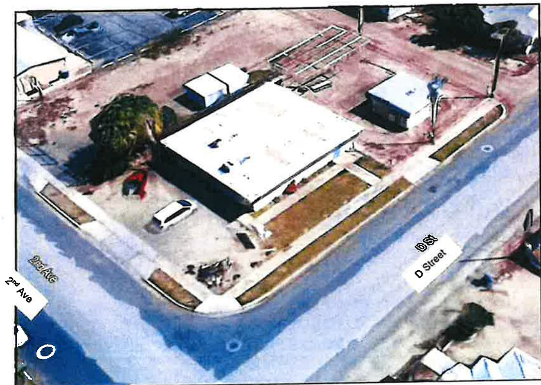
Figure 6 – Side and Top View of WCWD Administration Building
