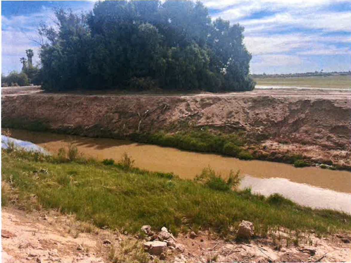
Photograph 4: Overview of the Central Drain Canal. View southeast, April 2, 2024.
