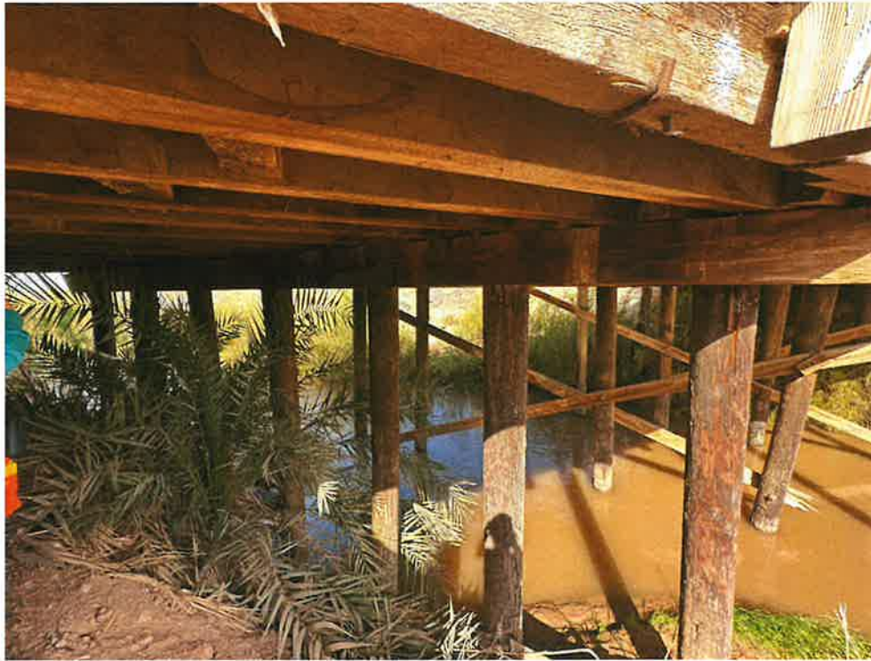
Photograph 3: Northwest-facing view from under Meloland Bridge.
