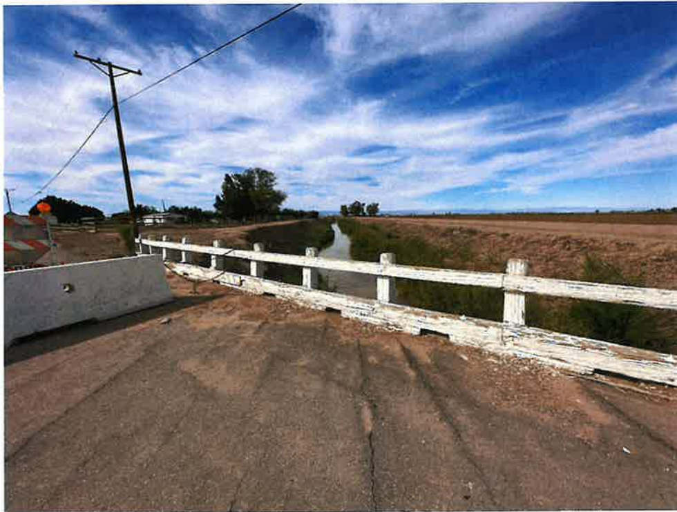
Photograph 5: Southwest-facing view from Meloland Bridge.
