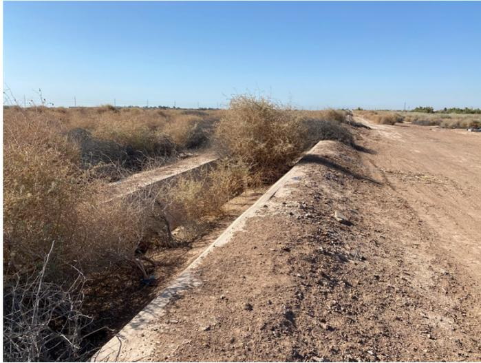
**Photograph 18** is located along the northern boundary of the Project, facing south. Photograph depicts Quailbush Scrub and an unused concrete-lined irrigation channel.
