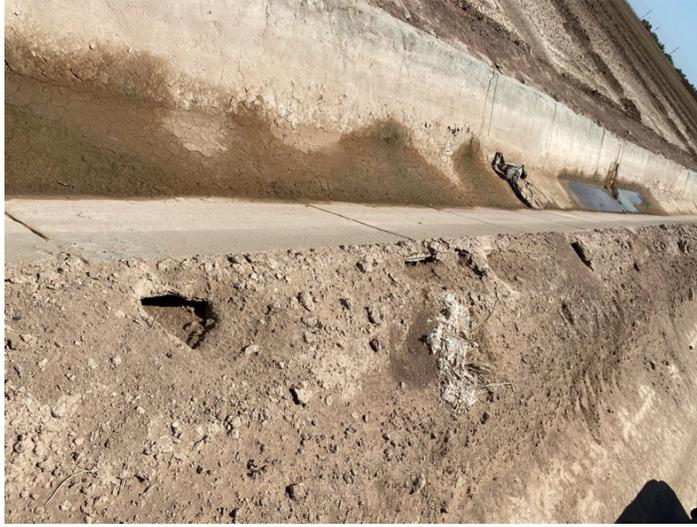
**Photograph 2** is located at the southern boundary Project site at the corner of Dahlia Lateral Eight, facing northeast. Photograph depicts erosion along edge of a concrete-lined irrigation channel that could potentially become burrowing owl burrows.
