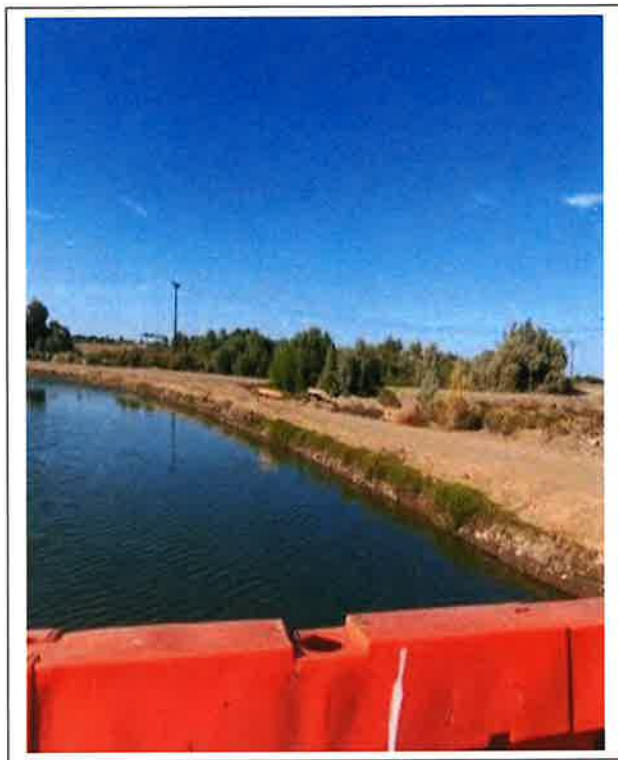
5. Facing south while on bridge 8/8
