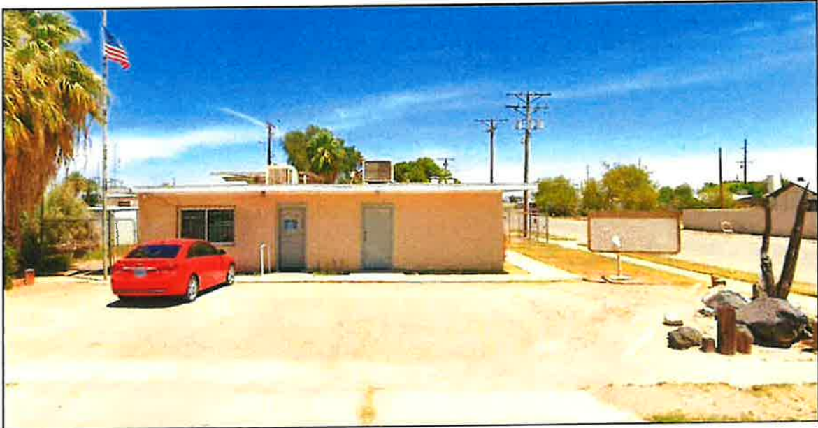
Figure 5 – Front View of WCWD Administration Building
