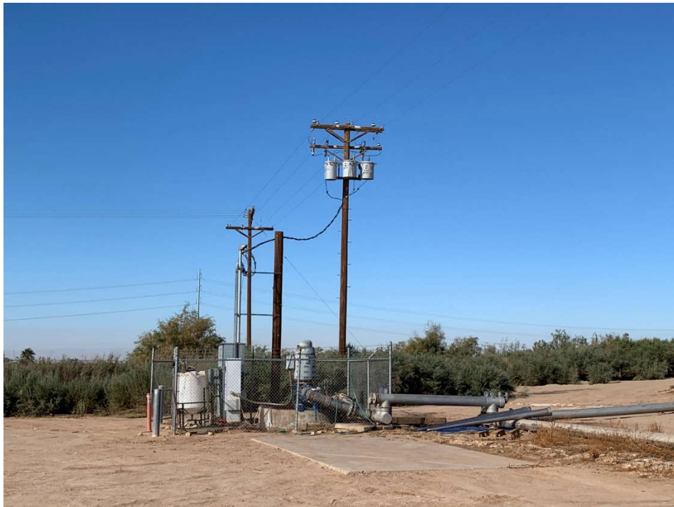
Photo 12: Looking west at the irrigation reservoir's pump system and pole mounted transformers within the north side of subject property east parcel from photo location #6 (Photo Location 6, Plate A-2).
