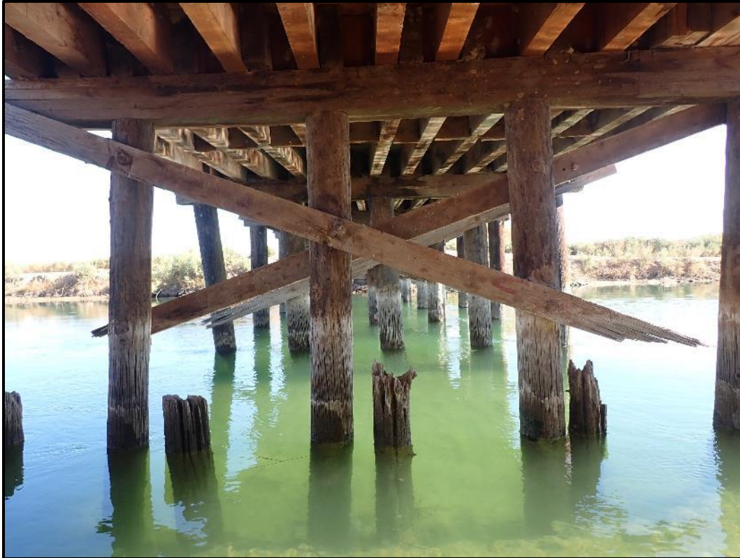
Figure 21. Detail of bridge construction, view to the west.
