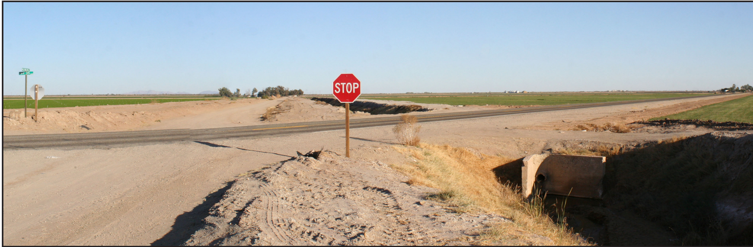
KOP 3: Evans Hewes Highway and Nelson Pit Road looking east - Existing Condition
