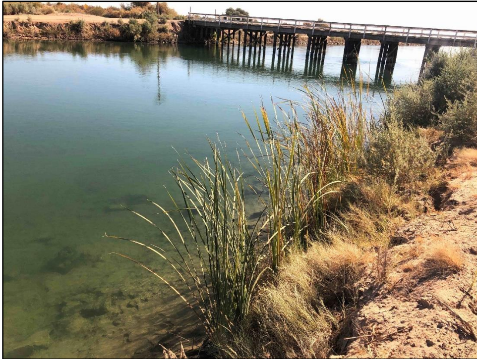
Photograph B-1. Vegetated banks of East Highline Canal, view facing southeast (upstream).
