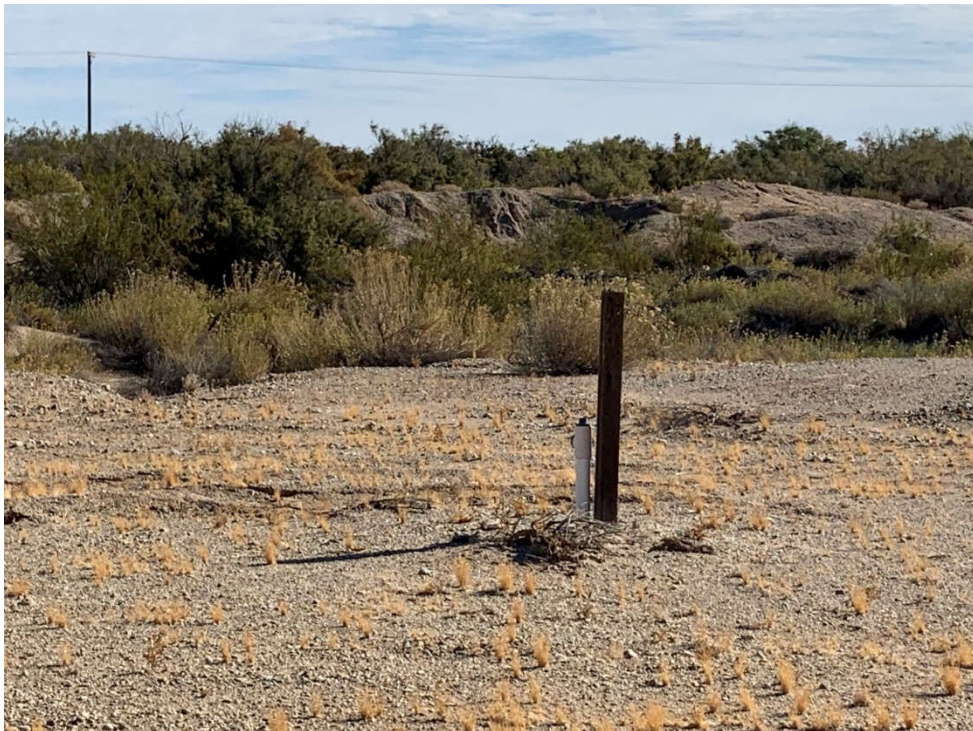
Photo 18: Looking east at water pipe within northwest parcel of the subject property (Photo Location 11, Plate A-2).
