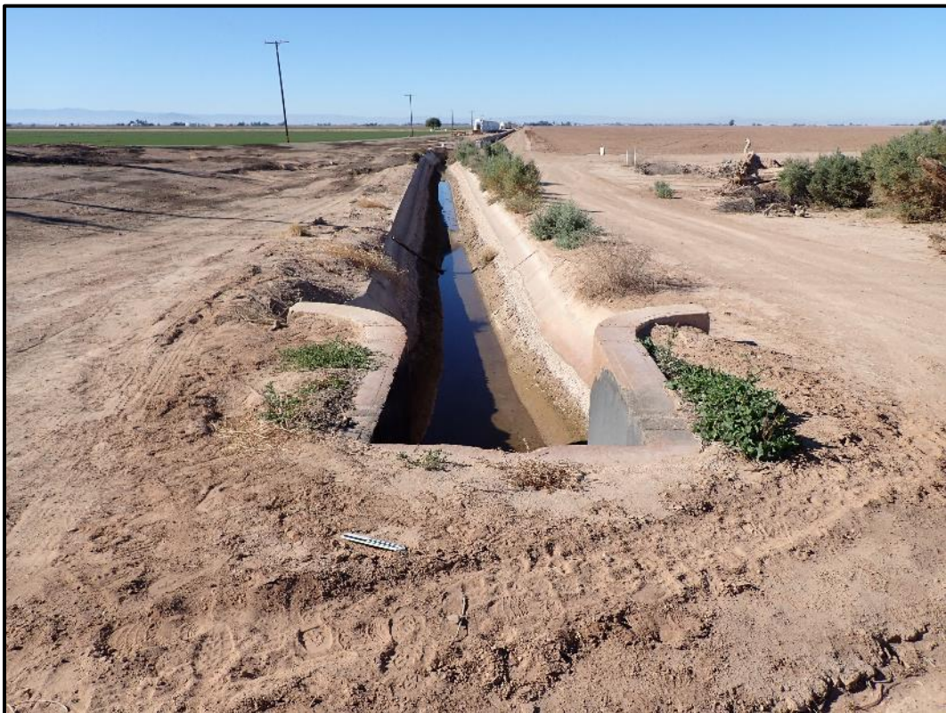
Figure 20. Overview of East Highline Canal, view to the west.
