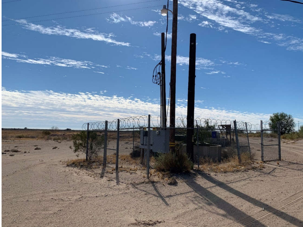
Photo 29: Looking south at cistern and pump south of shop within the eastern parcel of the subject property (Photo Location 17, Plate A-2).
