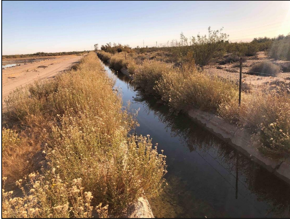
Photograph B-5. Concrete-lined channel East Lateral Eleven, view facing south (upstream).
