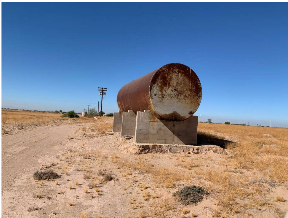
Photo 38: Looking west at large empty above ground tank and pole mounted transformers within the eastern parcel of the subject property (Photo Location 23, Plate A-2).
