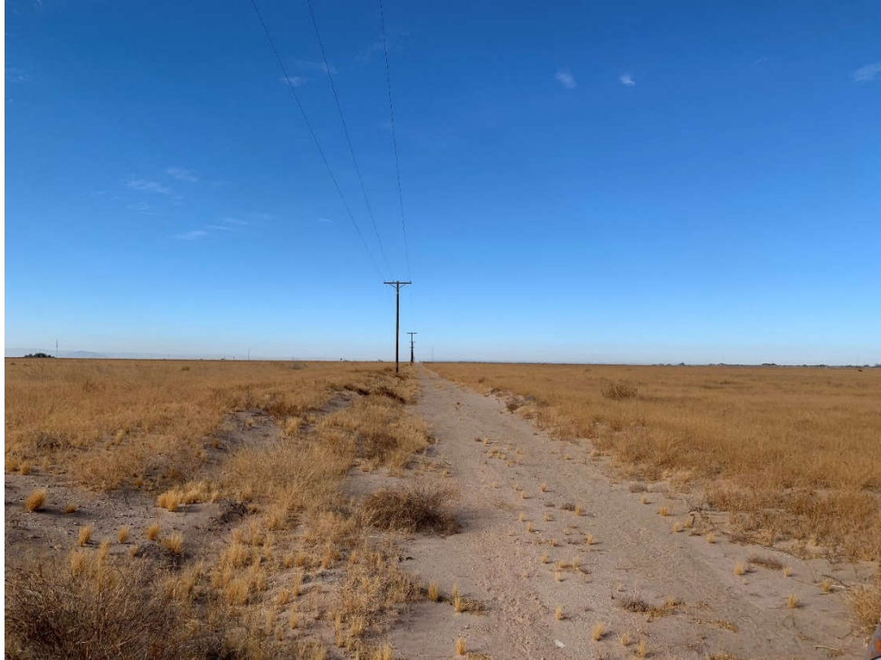
Photo 7: Looking west across the subject property east parcel from the east end of the field road at the north quarter of the site (Photo Location 3, Plate A-2).
