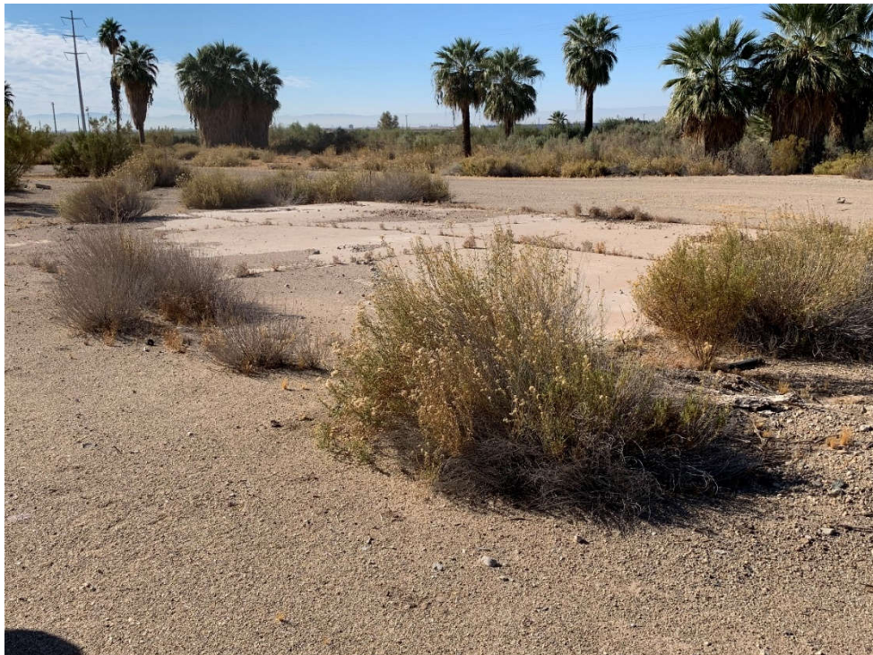
Photo 16: Looking southwest at concrete slab within northwest parcel of the subject property (Photo Location 10, Plate A-2).
