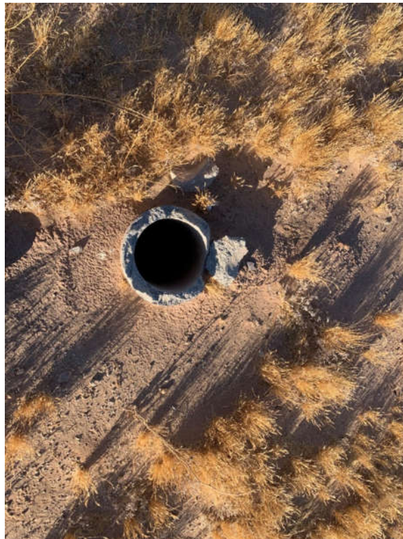
Photo 36: Looking at concrete transite water pipe remains within the eastern parcel of the subject property (Photo Location 22, Plate A-2).
