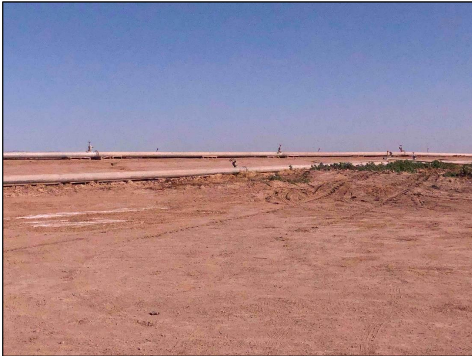
Photograph B-8. Irrigation pipe fed by East Highline Lateral Eleven used for watering adjacent croplands, view facing north.
