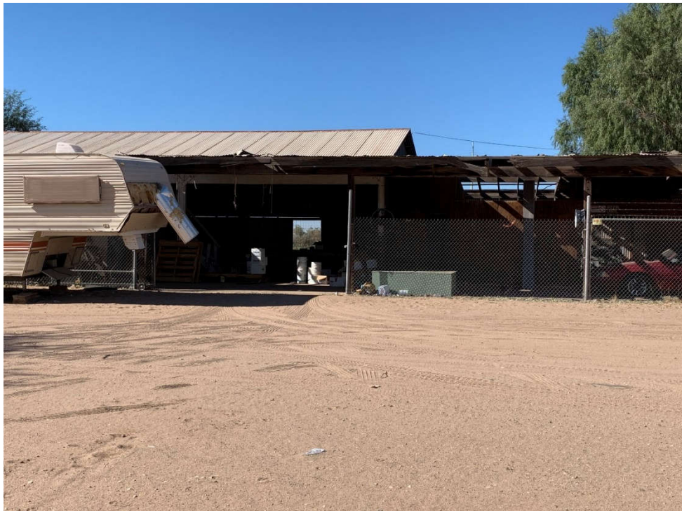
Photo 26: Looking west at the shop on the south side of the residence within the eastern parcel of the subject property (Photo Location 17, Plate A-2).
