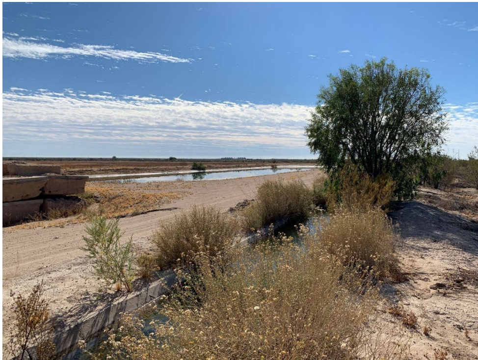
Photo 24: Looking southeast at the irrigation ditch and the reservoir at the southwest end of the eastern parcel of the subject property (Photo Location 15, Plate A-2).
