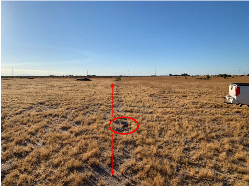
Photo 37: Looking at underground concrete transite water pipe within the eastern parcel of the subject property (Photo Location 22, Plate A-2).
