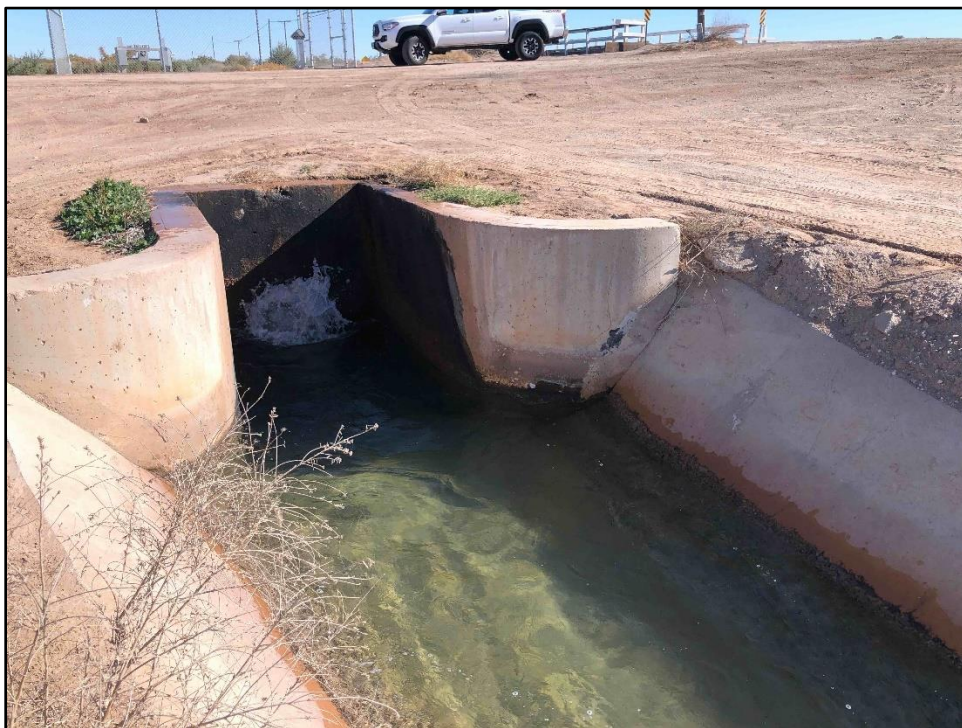
Photograph B-2. Pump feeding into East Highline Lateral Twelve, view facing east (upstream).
