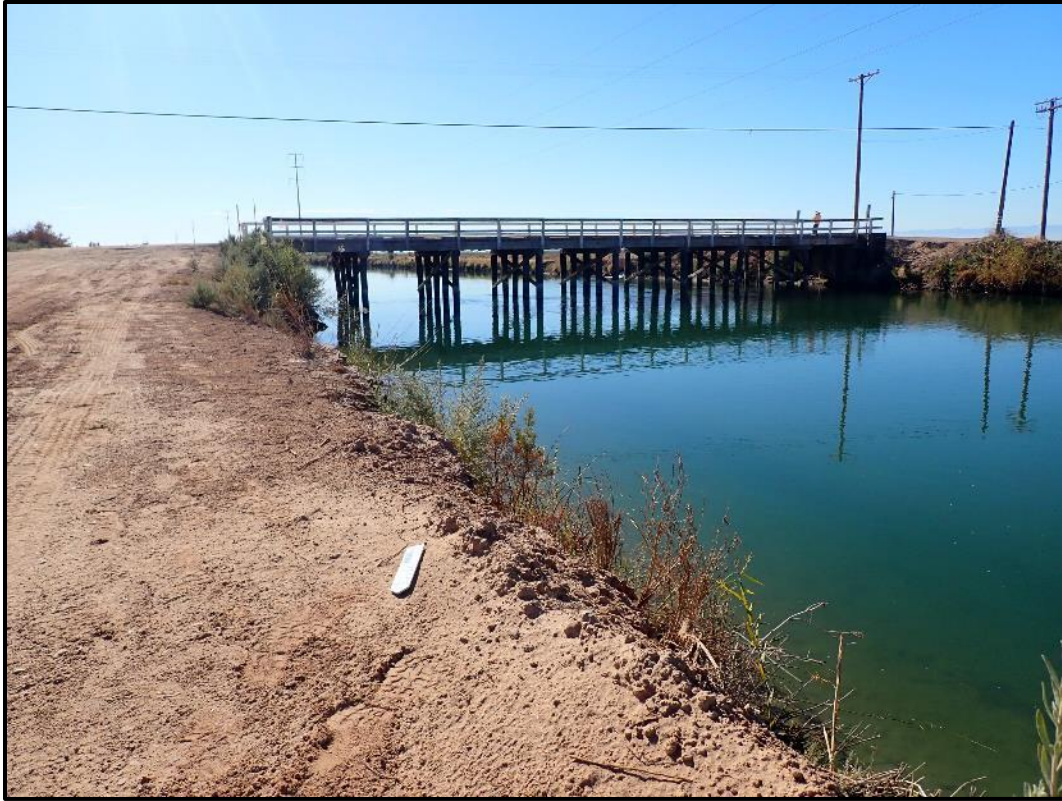
Figure 19. Overview of P-13/008333/CA-IMP-7835, view to the north.
