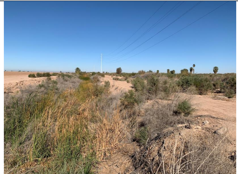
Figure 4. East Highline Canal Lateral Eleven north/south extension, between parcels 1 (to east; photo right) and 2 & 3 (viewing north).
