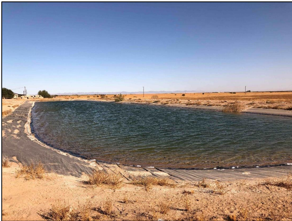
Photograph B-4. Geotextile lining along bank and inundated bed of Unnamed Reservoir 03, view facing northwest.
