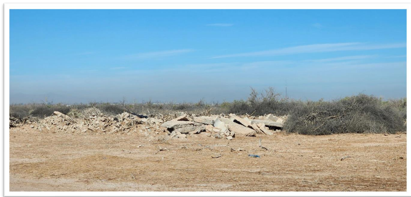
Photo 8: Northeast portion of the Project site with concrete rubble. View to the north.
