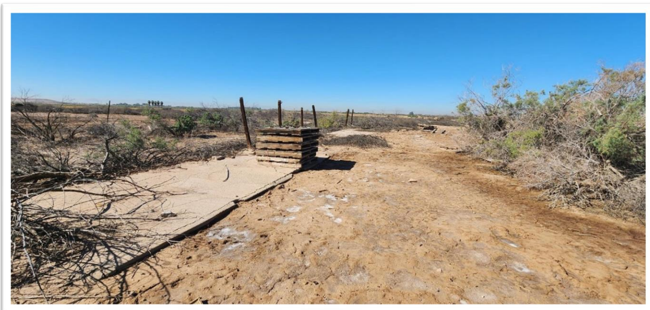
Photo 10: Northeast section of the Project site with concrete pad evident. View to the southwest.
