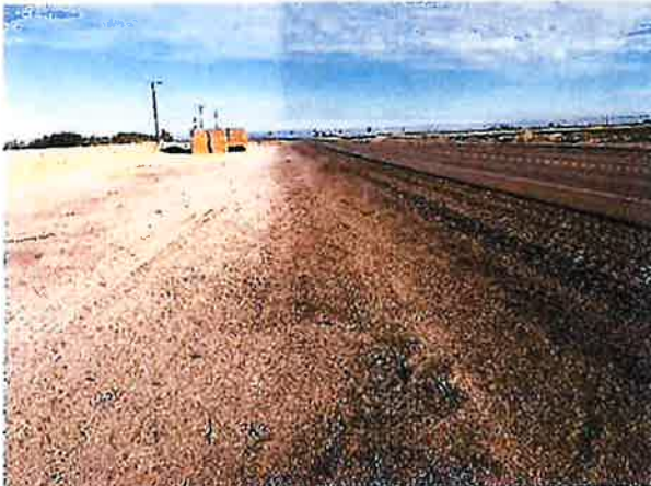
Photograph 5: Roadway to the south of the bridge.
