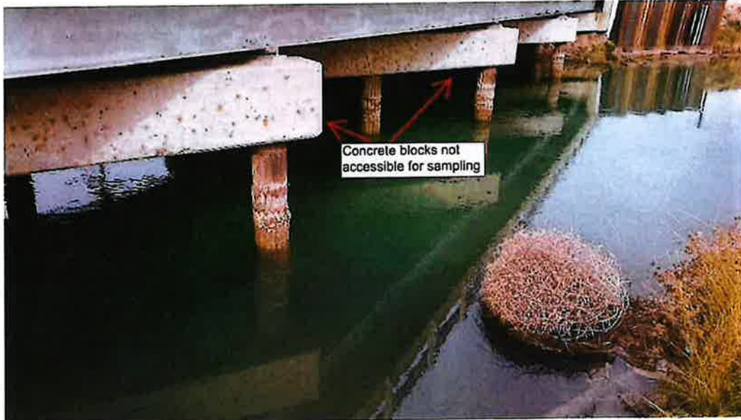
Photograph 12: Close-up of the concrete blocks beneath the bridge.
