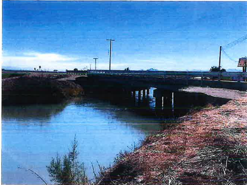
Figure 6. View of CA-IMP-7834, Westside Main Canal from the central portion of the survey coverage area facing south, also showing Bridge No. 58C-0114.
