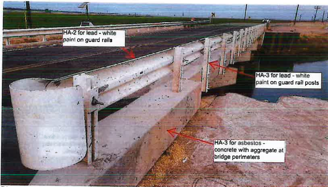
Photograph 15: Location of potential asbestos-containing material and potential lead-containing paint. Looking at the bridge from the southeast.
