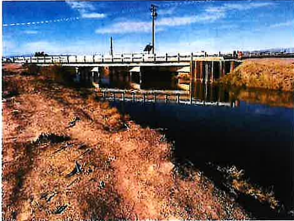
Photograph 3: Looking at the bridge from the east.
