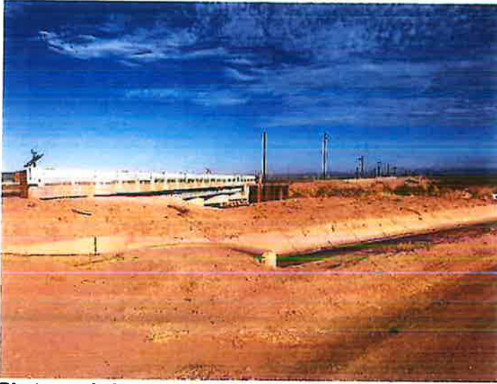
Photograph 1: Looking at the bridge from the southeast.
