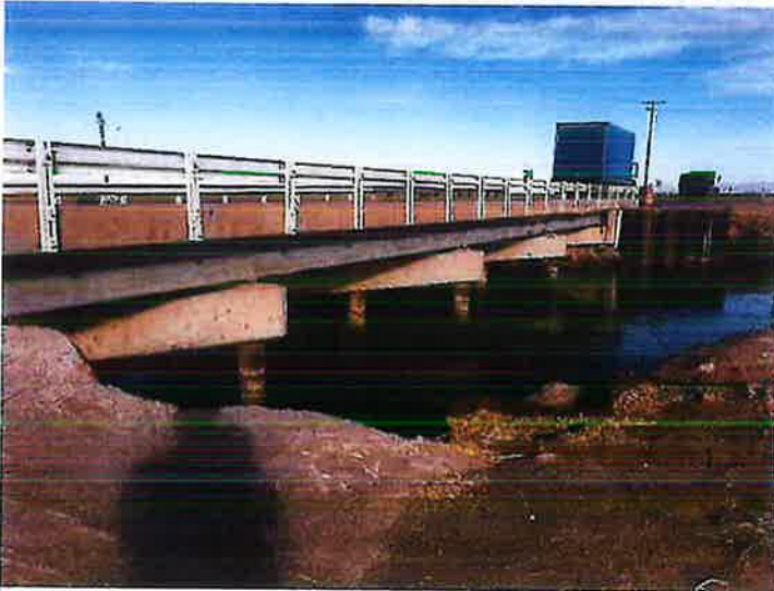
Photograph 2: Looking at the bridge from the southeast.
