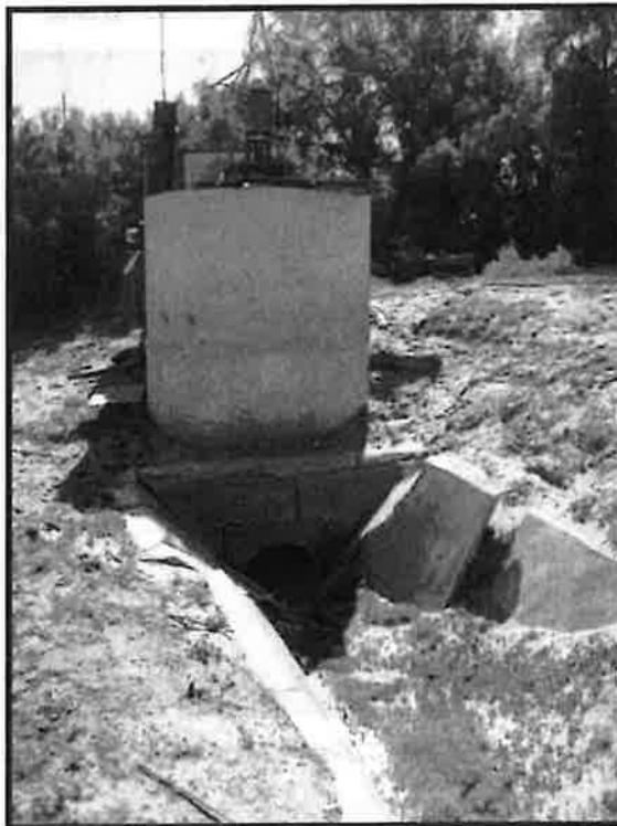
Looking south at the terminus and the north-south portion of WSM Pump 6
