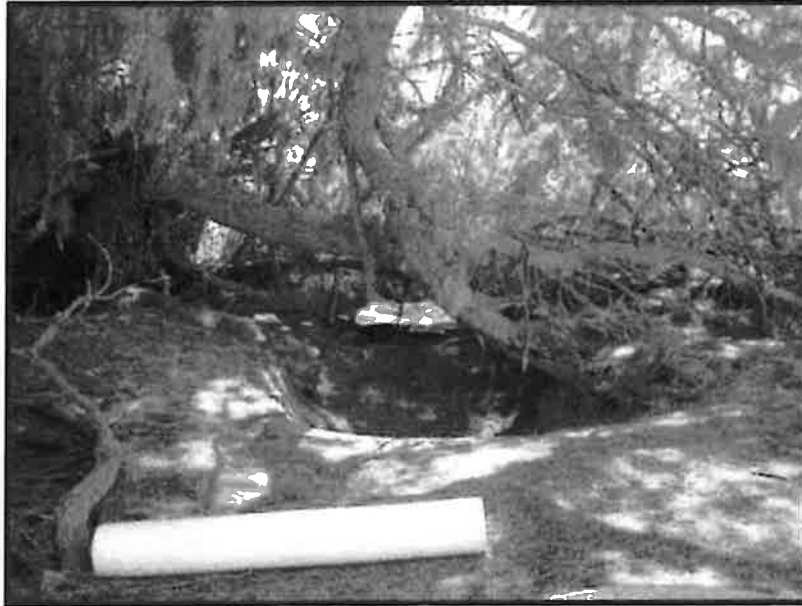
At the origin of the east-west portion looking south at concrete-lined structure
