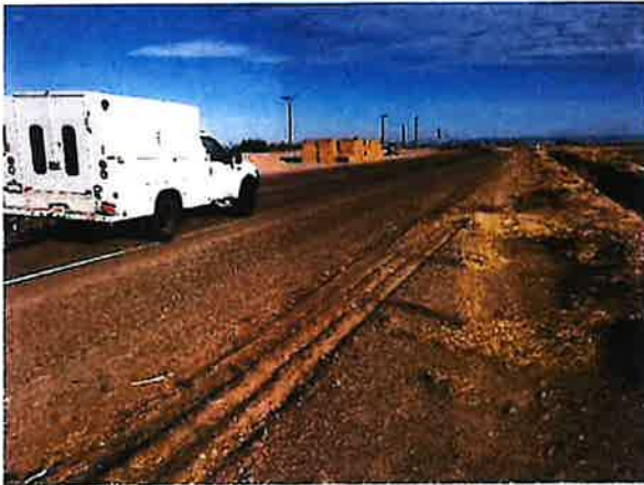
Photograph 4: Roadway to the south of the bridge.
