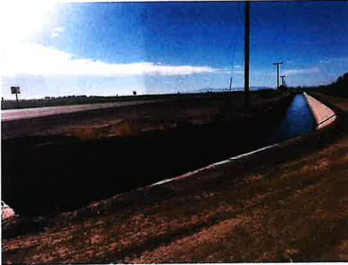
Photograph 8: Looking south at the Westside Canal.
