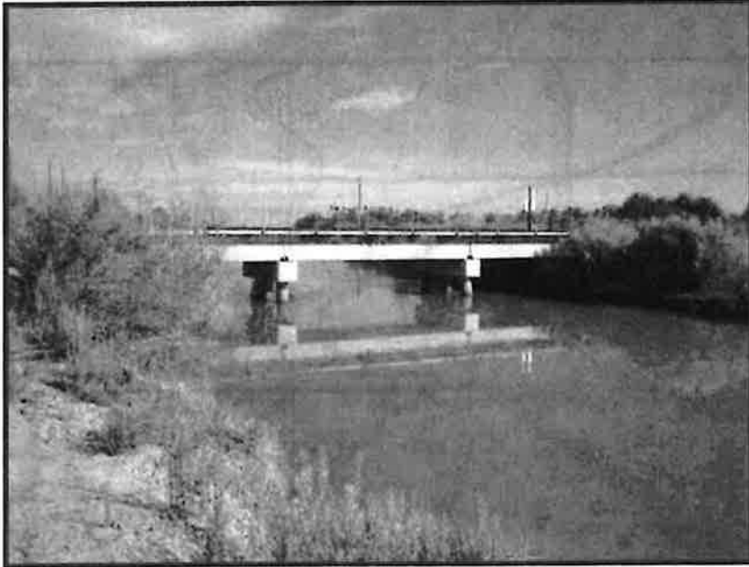
Westside Main Canal, SD- AZRR Crossing, View to the North
