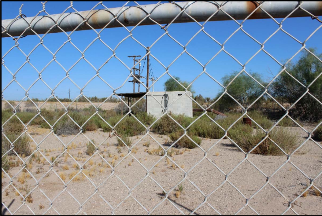
Photo 3: Masonry block pump house located at the north-central portion of the subject site.
