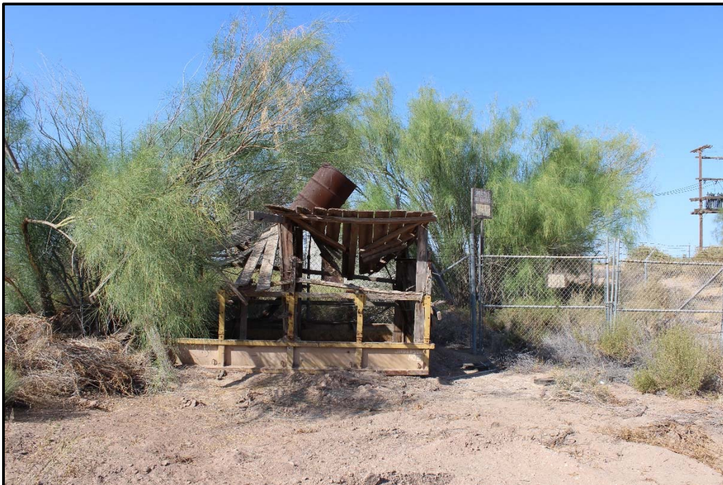
Photo 6: Miscellaneous building near farm yard.
