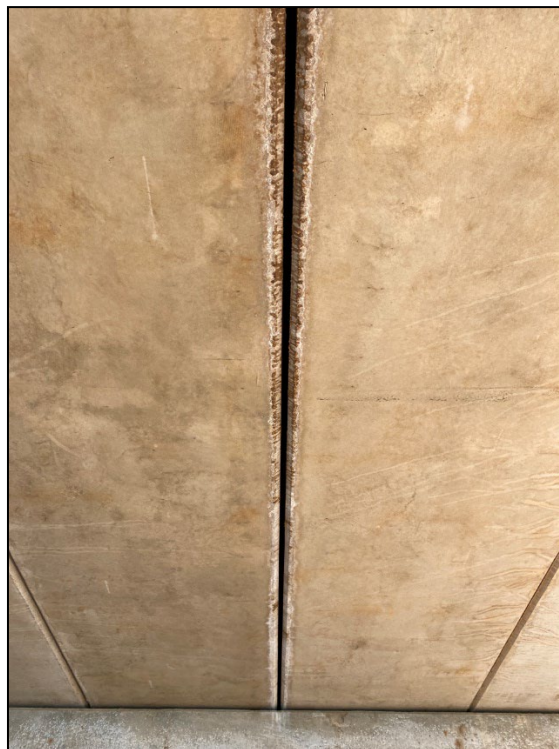
Photo 12. View of the crevice housing a bat colony within the Gordon Wells Road bridge crossing the offline storage canal for the All-American Canal.
