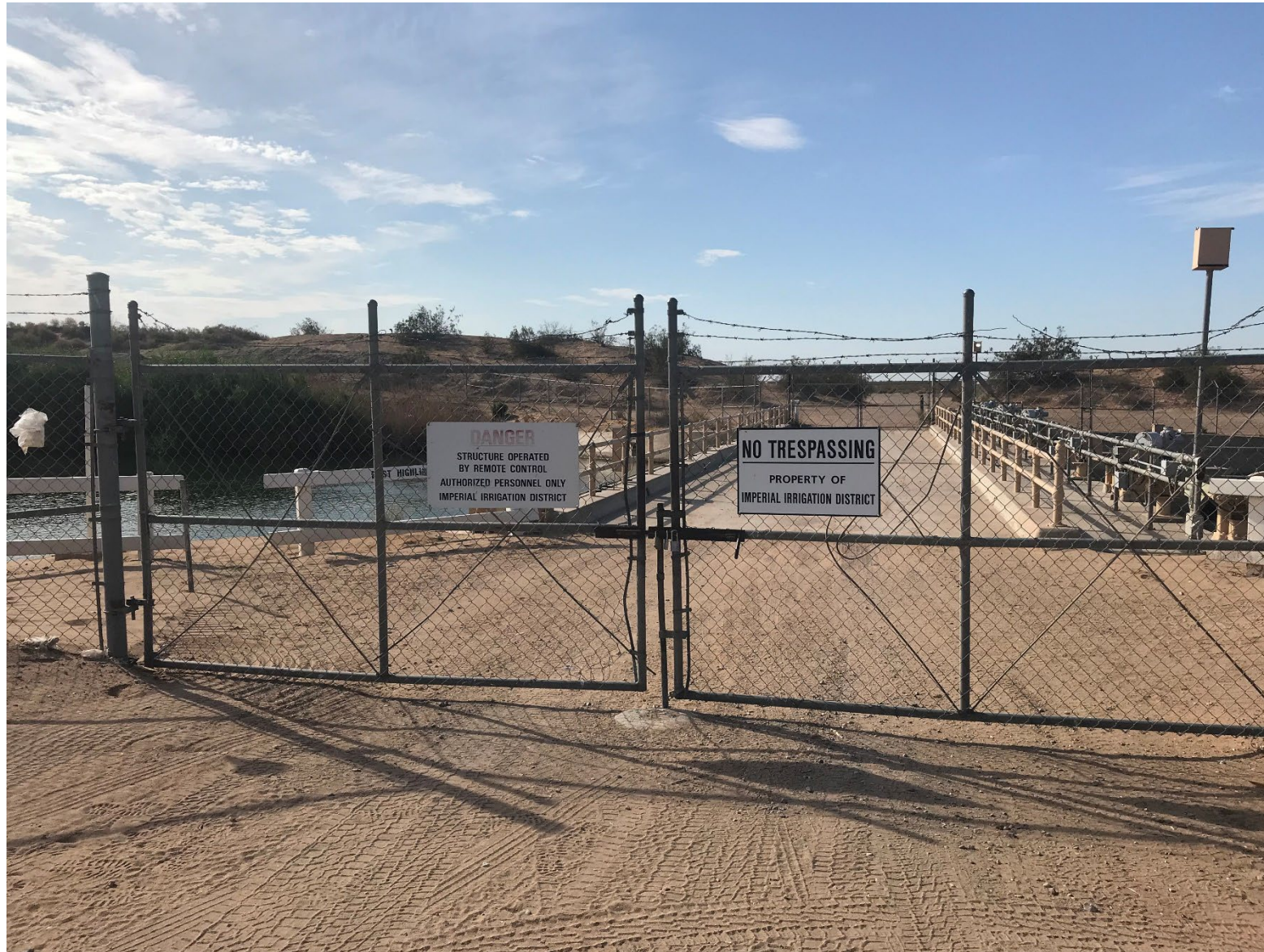
Figure 2-5. Bridge Crossing – Pedestrian Access Only
