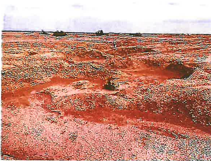
Photo 2: Drainage 1 where a bed, bank, and channel begin to develop within the Impact Area of proposed well pad 18-32 (at RA 1D) after being partially diverted by Drainage 2 at RA 2. Photo taken facing east along the southern edge of the access road Impact Area on April 26, 2022.
