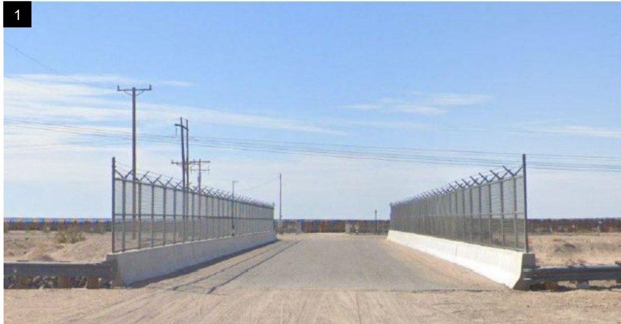
Bridge over north American Canal
