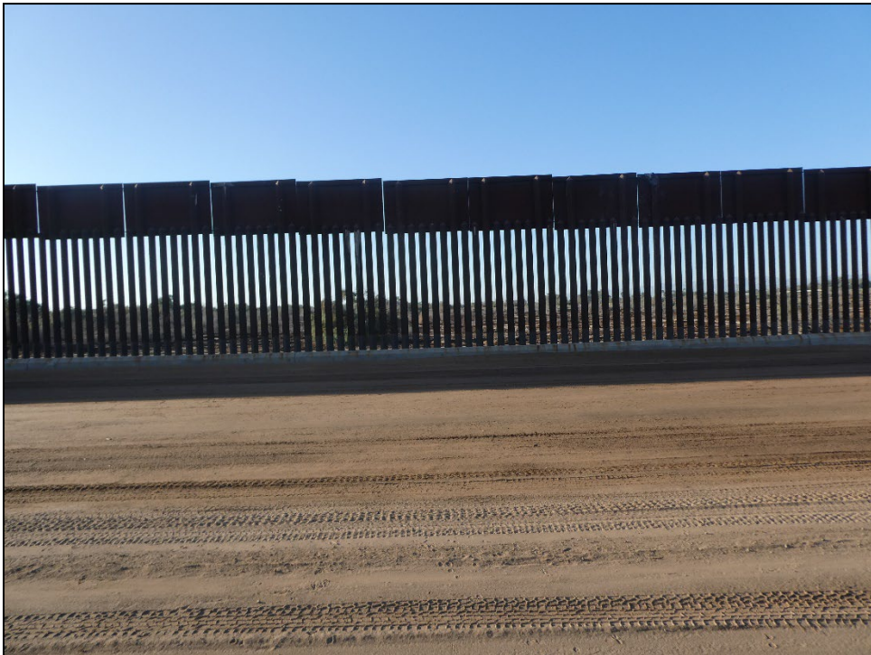
Photo 8. View of U.S. Mexico border wall lining the southern perimeter of the Project Area, facing south.
