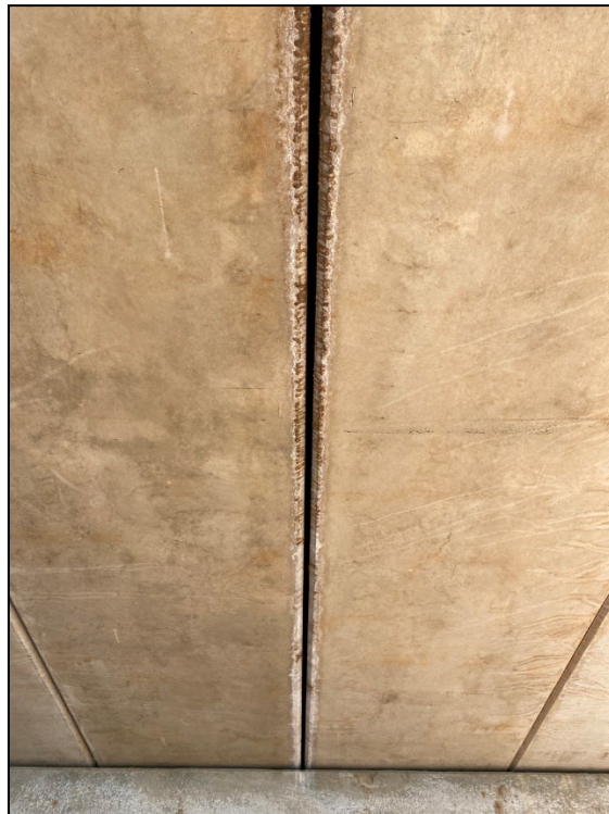
Photo 12. View of the crevice housing a bat colony within the Gordon Wells Road bridge crossing the offline storage canal for the All-American Canal.
