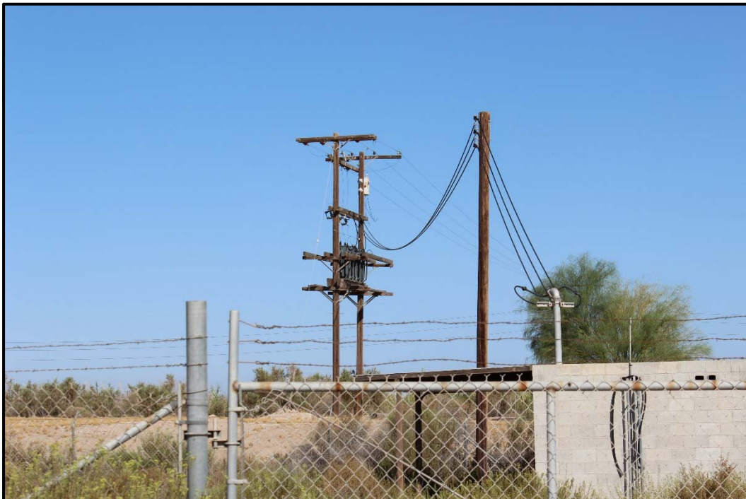
Photo 4: Clos-up view of pump house and transformer bank.
