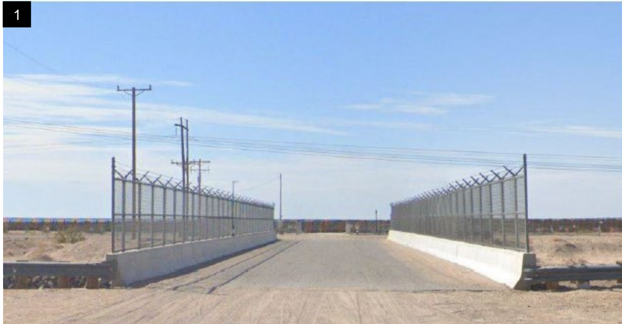
Bridge over north American Canal
