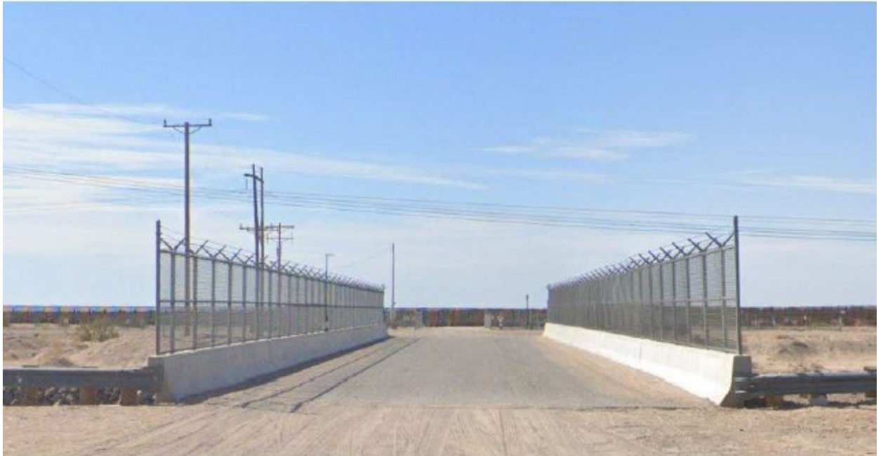
Bridge over north American Canal
