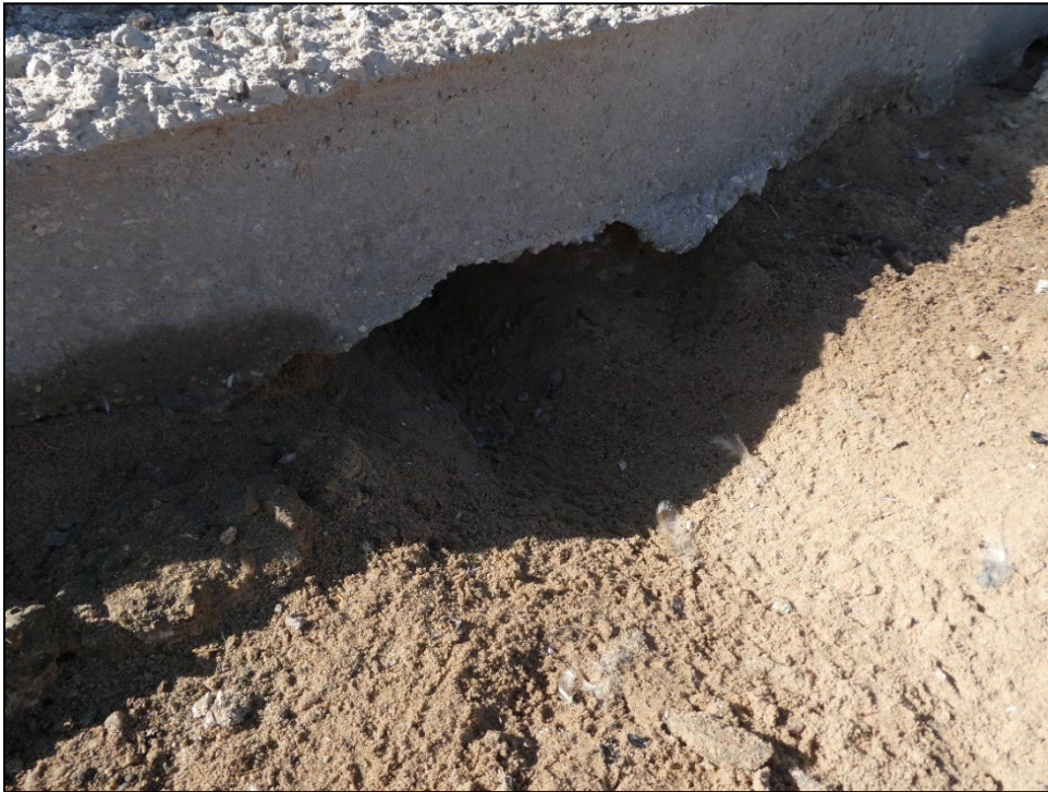
Photo 6. Close-up view of active burrowing owl burrow with whitewash and pellets near entrance, located in the southwestern section of the Project Area, facing southwest.
