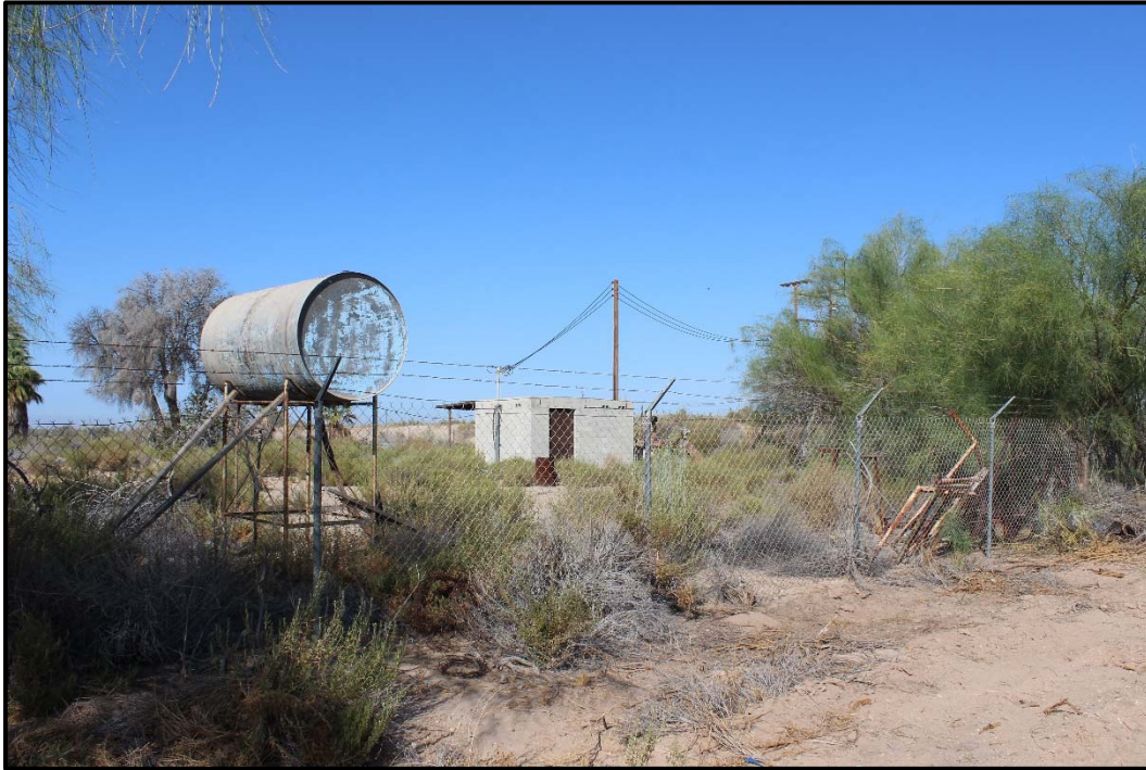
Photo 5: Above ground fuel tank (AST) within farm yard.
