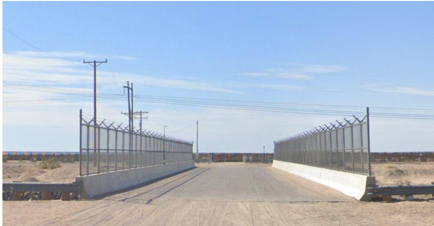
Bridge over north American Canal
