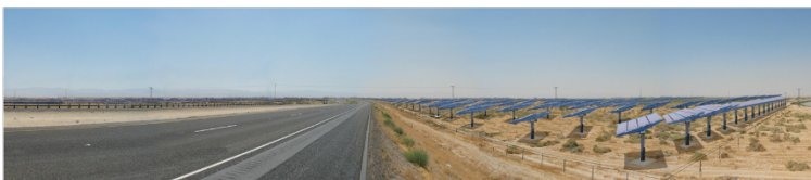
Visual Panoramic Simulation - View of Solar Energy Facility Site CPV panels and on-site transmission line towers
