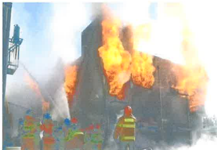
One of South Korea's big batteries having a 'moment'
