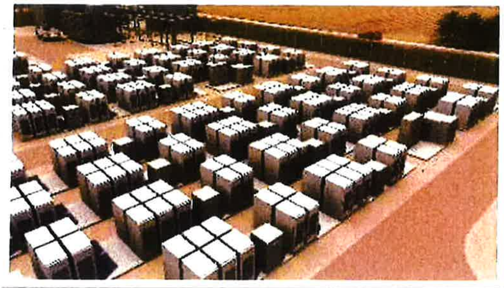
Modular ESS Installed on Multiple Concrete Pads
