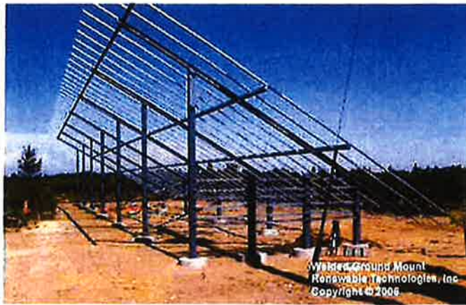
Typical fixed tilt mounting structure
