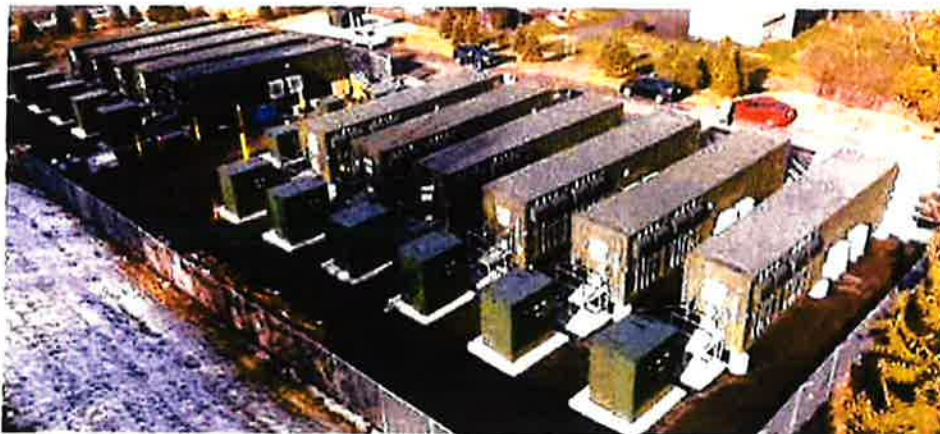
Modular ESS Installed on Concrete Pad
