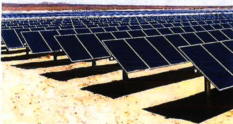
Typical single axis tracking solar panels
