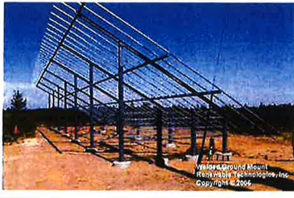
Typical fixed tilt mounting structure
