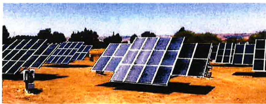
Typical dual axis tracking solar panels
