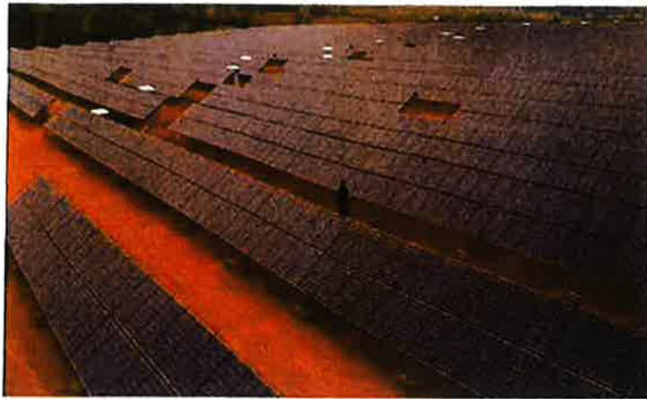
Typical fixed-tilt solar panel rows
