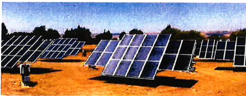
Typical dual axis tracking solar panels
