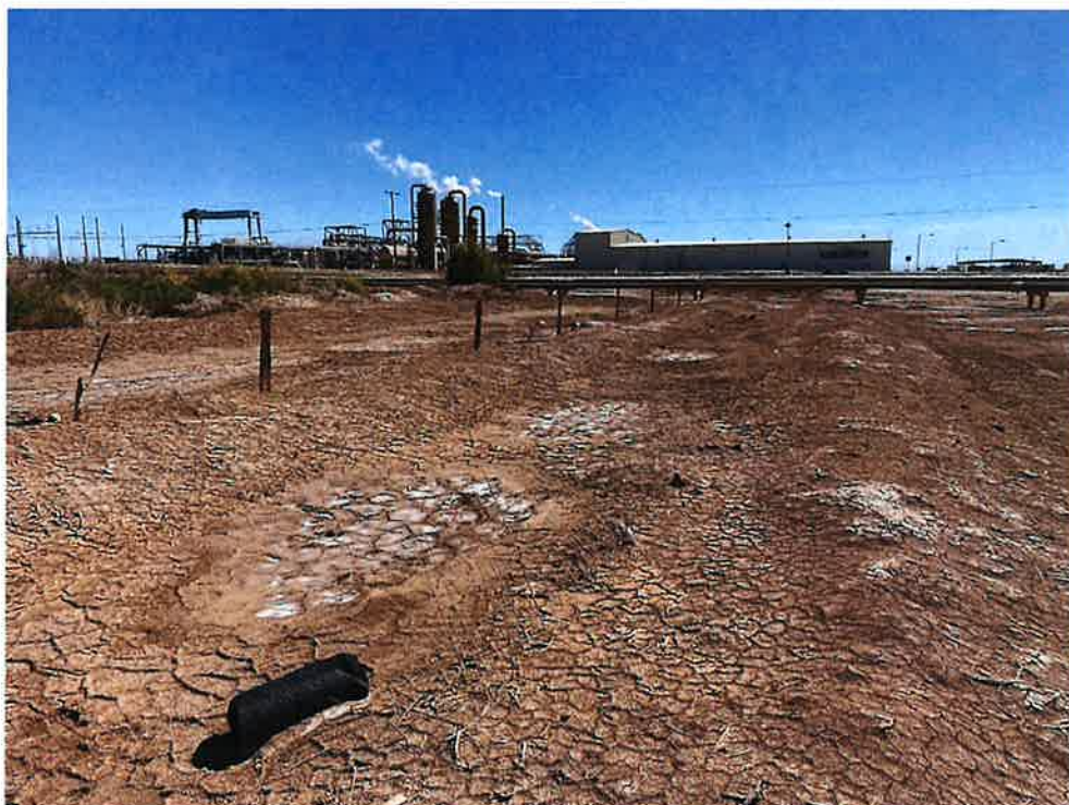
Figure 5. View from the southern portion of the project area, facing south to the existing geothermal plant.
