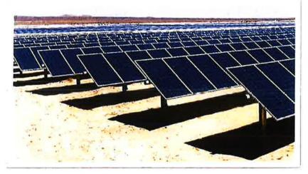
Typical single axis tracking solar panels
