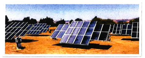
Typical dual axis tracking solar panels
