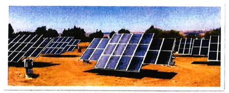
Typical dual axis tracking solar panels
