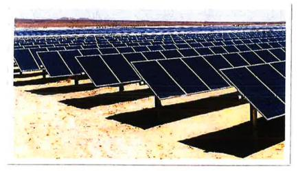
Typical single axis tracking solar panels
