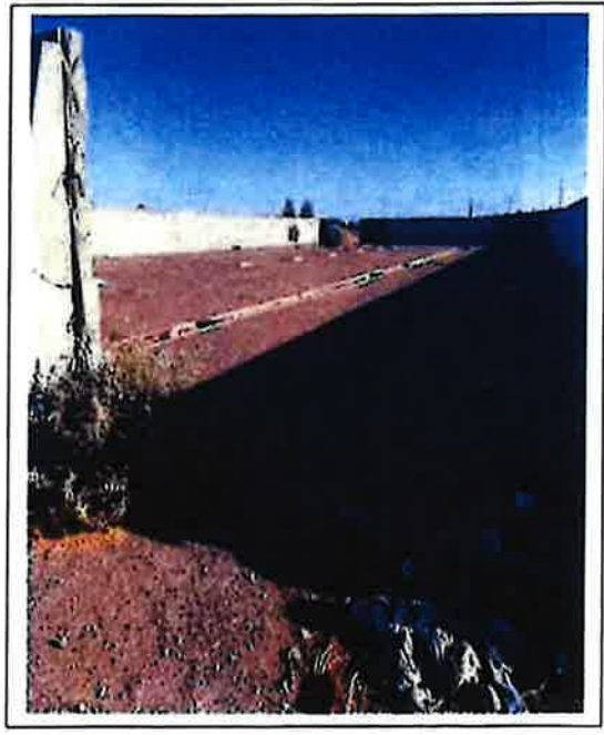
4. Inside area of concrete structure; quailbush in foreground
