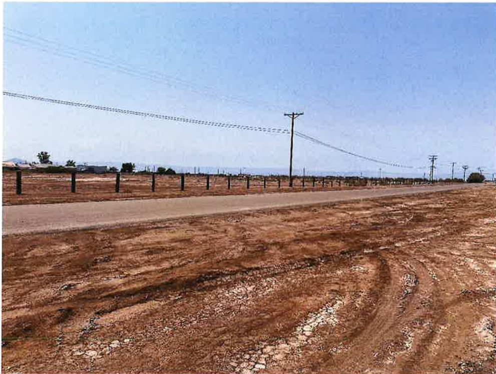
Belford Facing West
