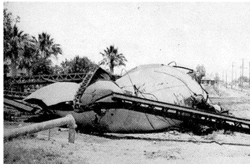
Figure 26. City of Imperial: Collapse of Walls and the 100,000-Gallon Water Tank (Photos: USCGS)
