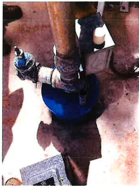
Photograph 7 - RV Park Well 1 (1)
