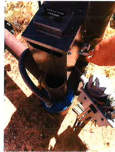
Photograph 12 - RV Park Well 3 (2)
