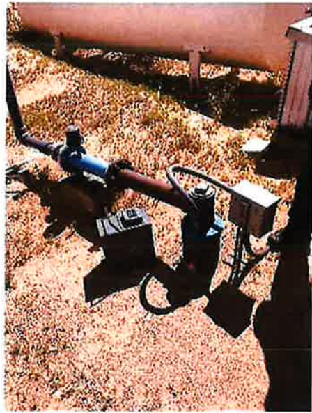
Photograph 11 - RV Park Well 3 (1)
