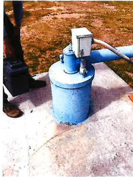
Photograph 10 - RV Park Well 2 (2)
