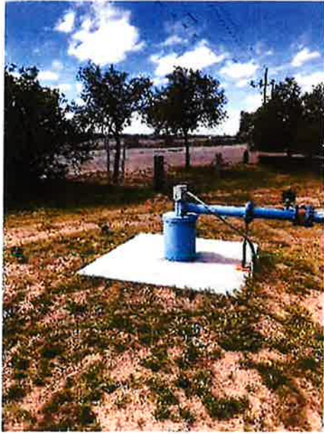
Photograph 9 - RV Park Well 2 (1)
