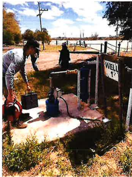
Photograph 8 - RV Park Well 1 (2)
