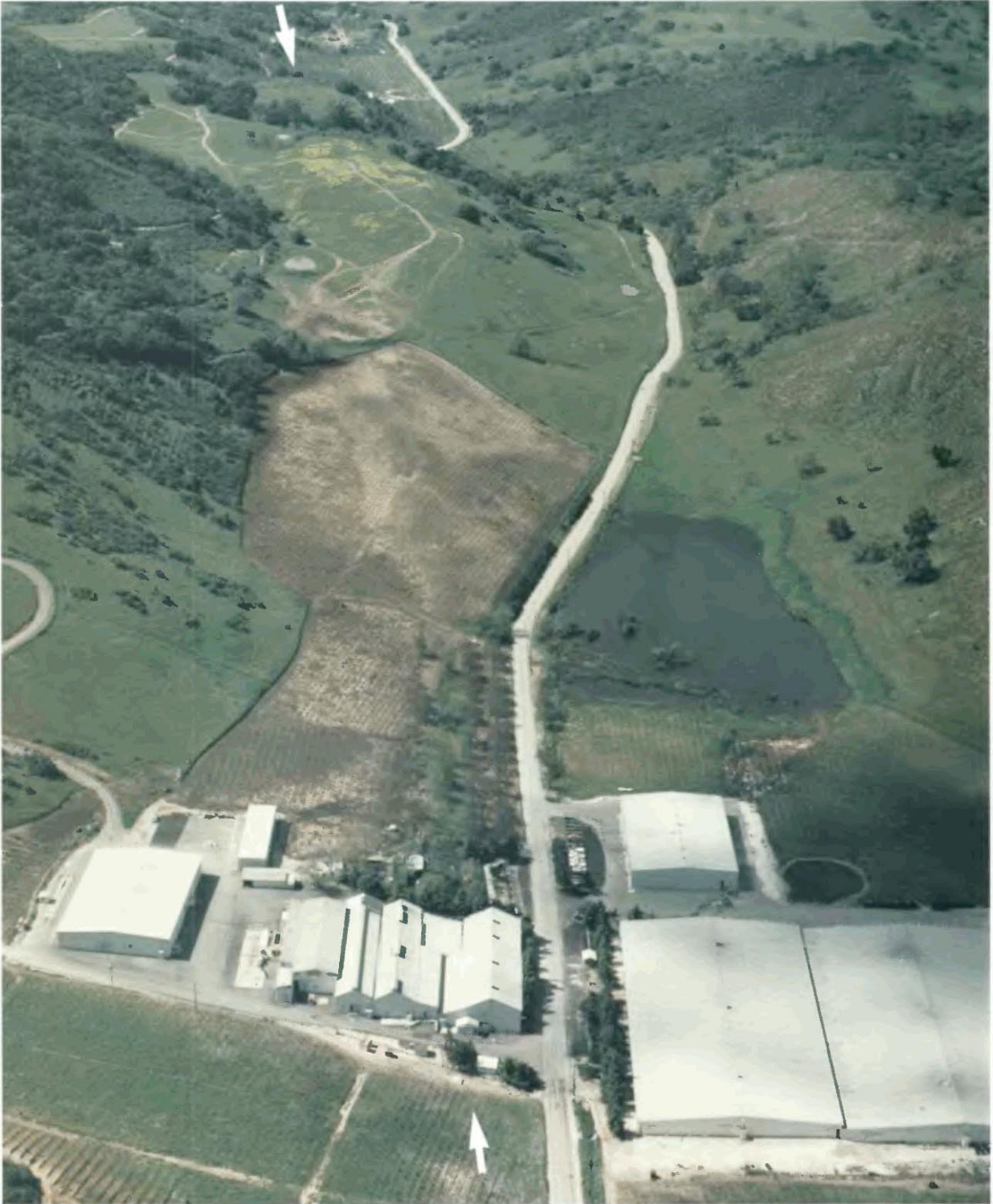
FIGURE 2.14.—Fault creep on the San Andreas fault was first reported at the Paicines Winery south of San Juan Bautista in 1960 by Steinbrugge and Zacher (1960). Fault trace (between arrows) passes under winery building, and walls of building are continually being displaced. View northwestward.
