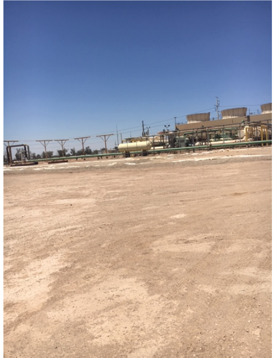
Photo 6 – central portion of development site.
