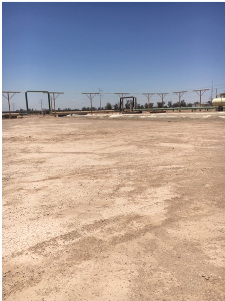
Photo 5 – central portion of development site.
