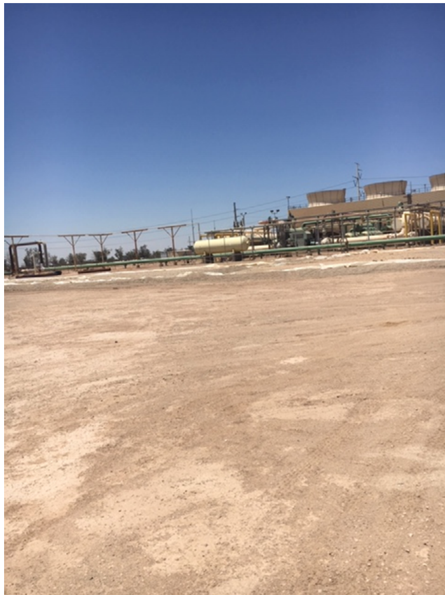
Photo 6 – central portion of development site.
