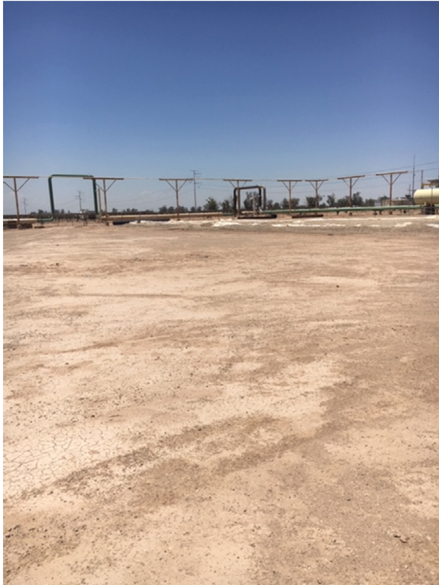
Photo 5 – central portion of development site.
