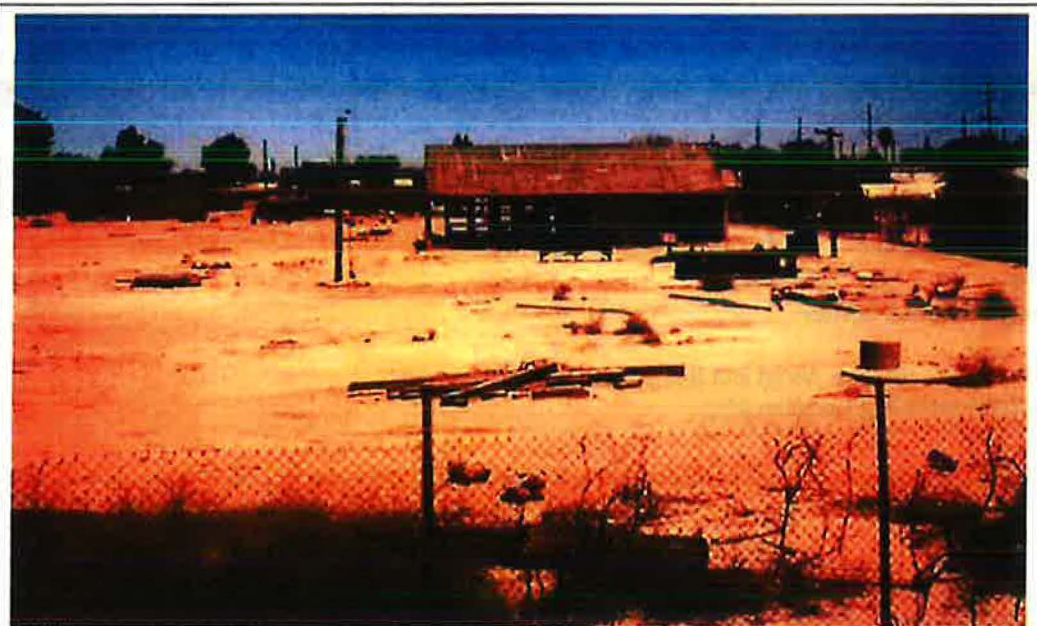
View north from Evan Hewes Highway towards project parcel. Existing structure will have to be demolished. Scattered debris and vegetation will have to be removed.
