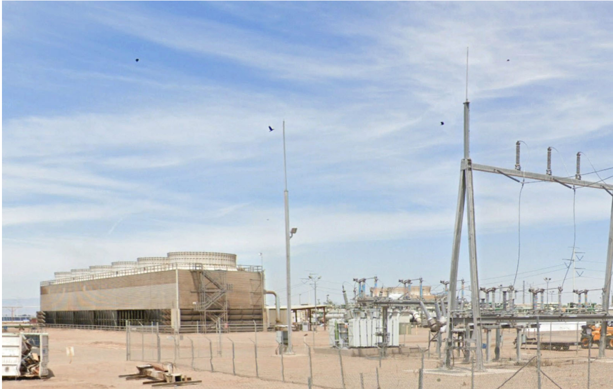
Photo 2. Four common ravens leaving the project site. Photo by Google Earth StreetView.
