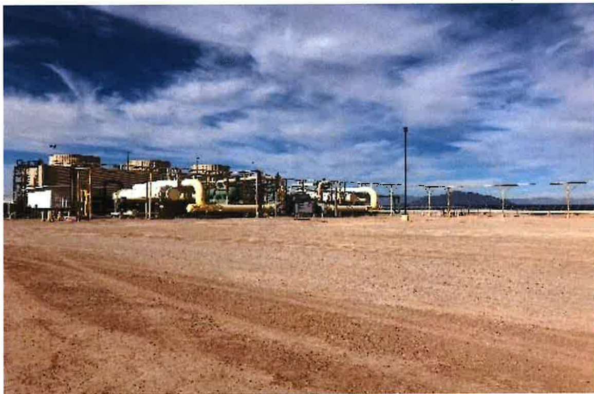
Figure 6- Photo of Project Site (June 13, 2019)
