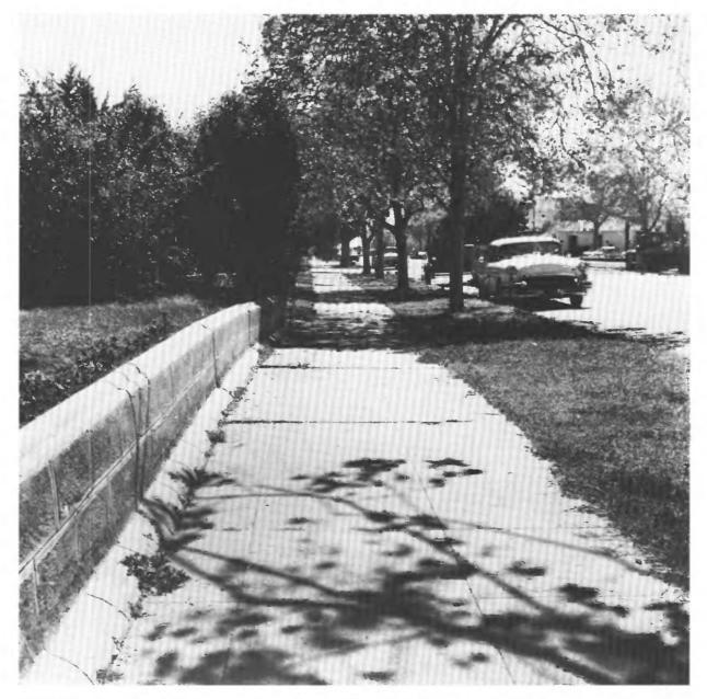
FIGURE 2.36.—Creep of about 1 cm/yr on the Calaveras fault in Hollister, Calif., has bowed walls, sidewalks, streets, and houses. View eastward at Sixth Street.
