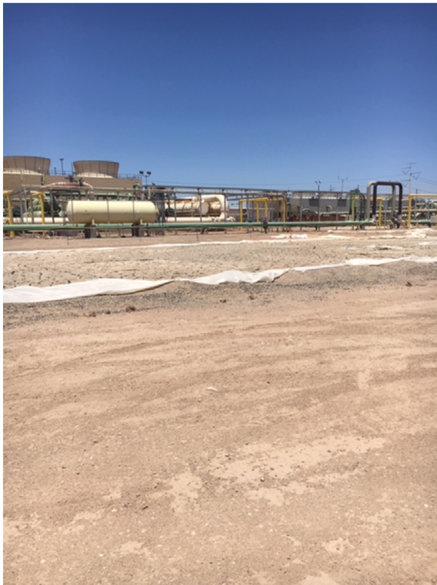
Photo 7 – northern portion of development site.
