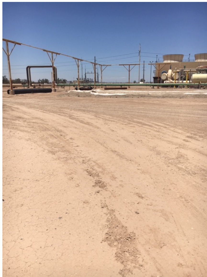
Photo 4 – northern portion of development site.
