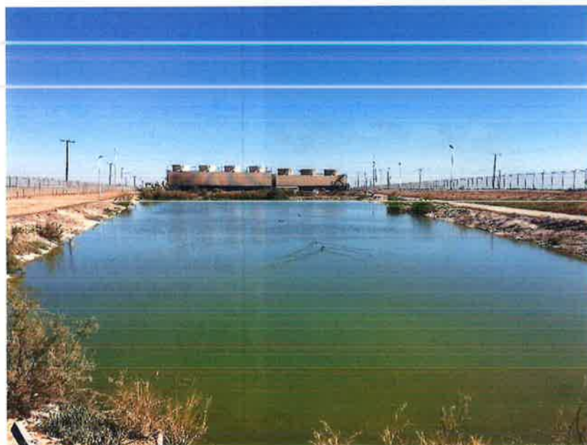
Photo 4. Overview of areas of the existing retention ponds (Open Water), Disturbed habitat surrounding the ponds, and existing cooling towers in the background. View north.
