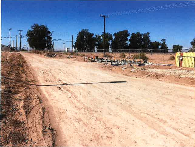
Photo 1. Overview of a typical access road along the western edge of the Study Area. View south.
