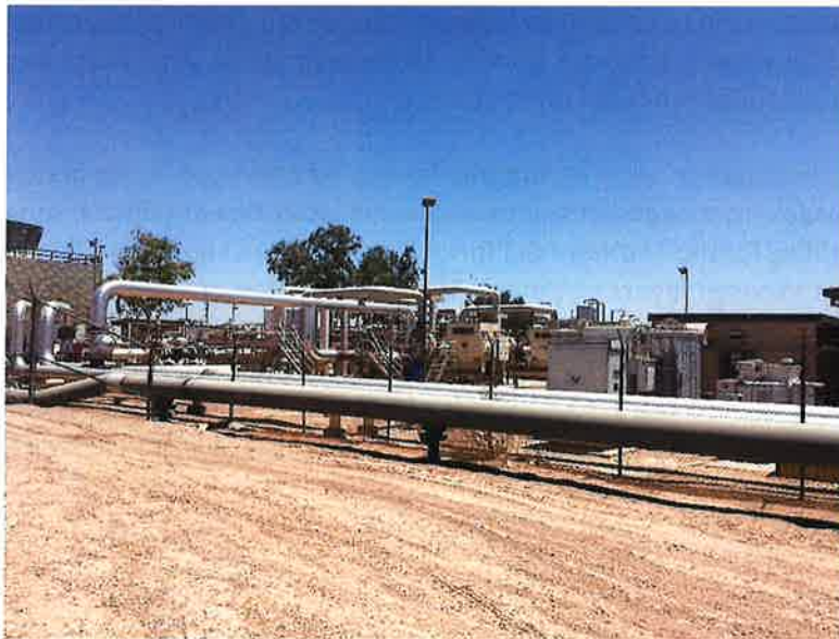
Figure 2: Overview of Project Area, facing southeast.
