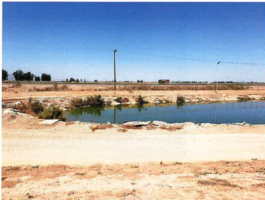
Photograph 2: View of the south end of the existing ponds.
