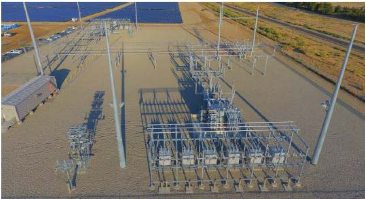
Figure 3-5. Representative Example of Typical Substation Design
