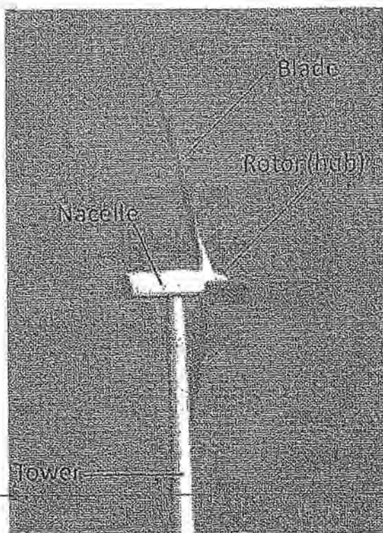
Major components of a modern wind turbine
