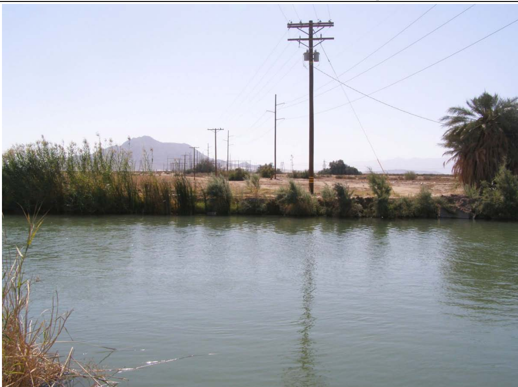
Figure 5. Viewshed from the Westside Main Canal at Leibert Road., looking south towards Imperial Valley Substation.
