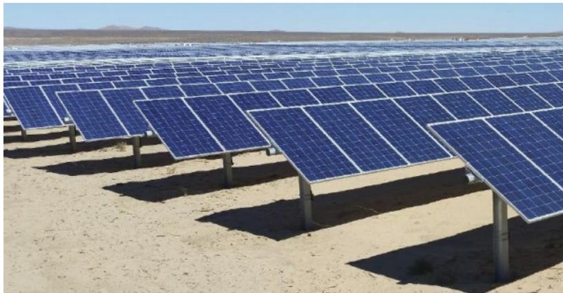
**Typical Single-Axis Tracking Solar Panels**
