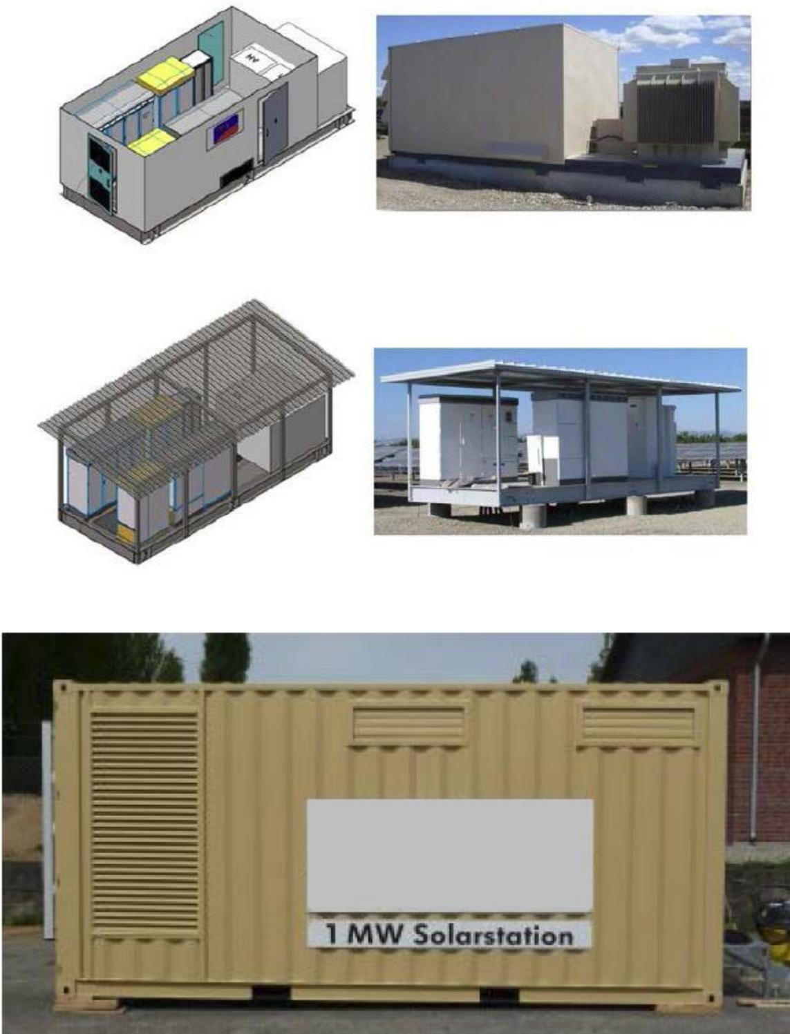
**Figure 3-6. Representative Example of Typical Substation Design**
